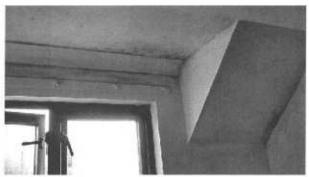
Photo 3: drying area – the condensation problem would be alleviated if tenants used drying area outside the flat. The landlord will check that the tumble drier is working.
