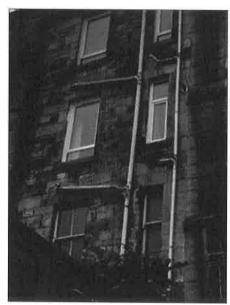
Seal between the original stonework and the double-glazed unit has been filled with expandable foam and white silicon. Window is now fully sealed and wind and water tight.
