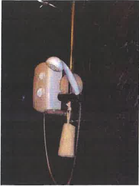
3. Repaired shower head/riser.
