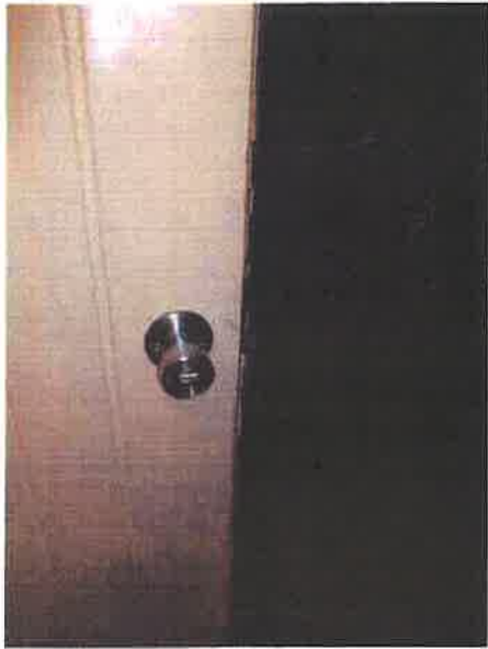
7. Bathroom door and panelling.
