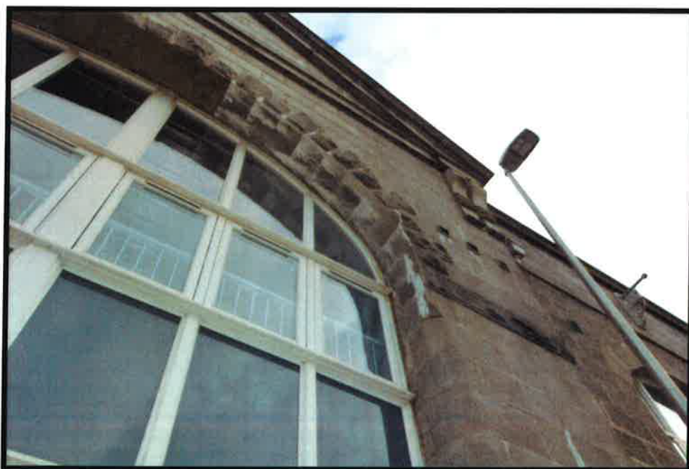
Photograph 7 Front elevation - Efflorescence to arched window masonry, as before.
