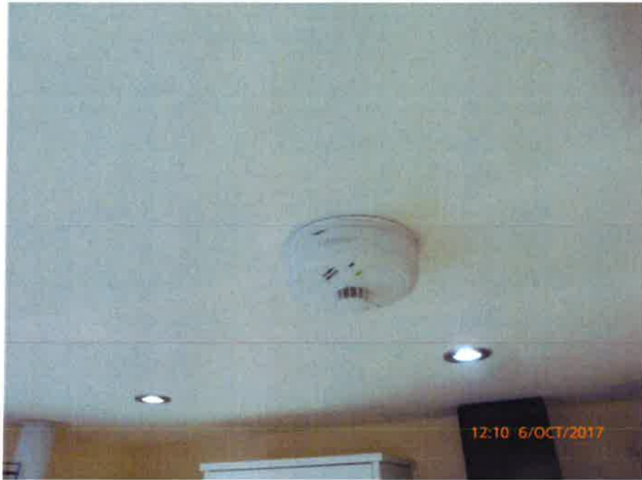
Heat detector in the kitchen
