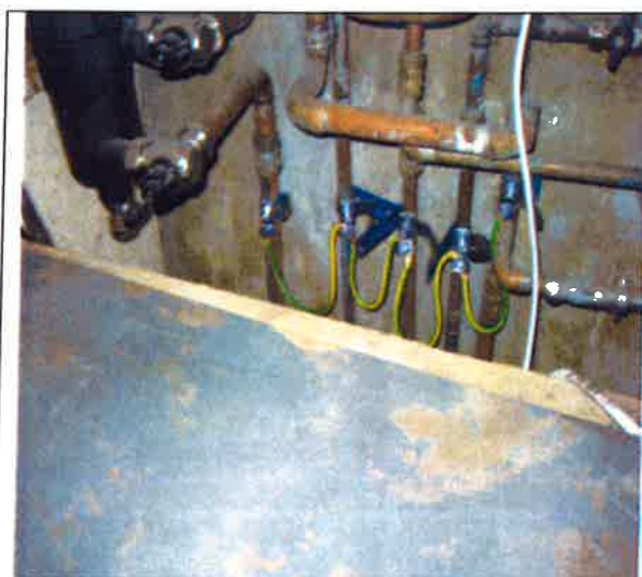
Bonding to gas pipes at boiler
