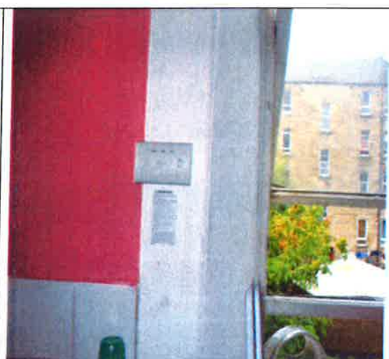
Carbon monoxide detector beside boiler
