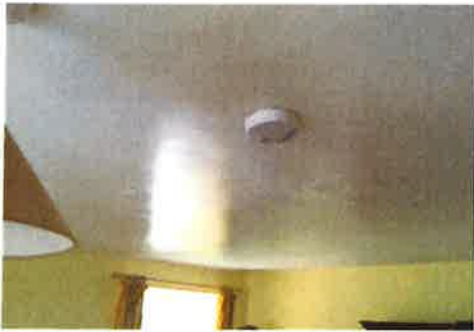
Upper floor battery operated smoke alarm 28-08-17
