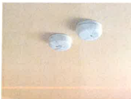
Ground Floor Replacement hard wired smoke alarm & heat detector 08-11-17
