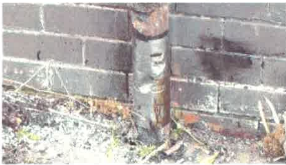
Photo 4 – Patched downpipe
