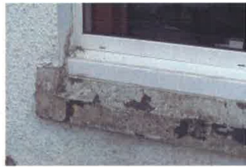
Photo 5 – Sill closing strip
