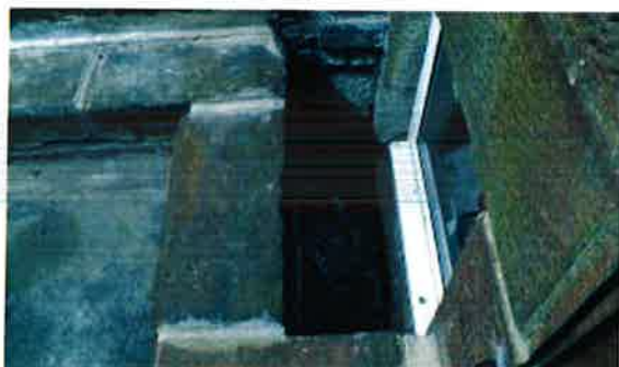
Photo 3 – External sill and soakaway
