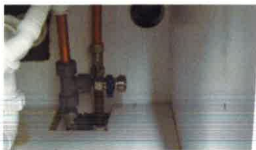
Photo 4 – Washing machine pipework
