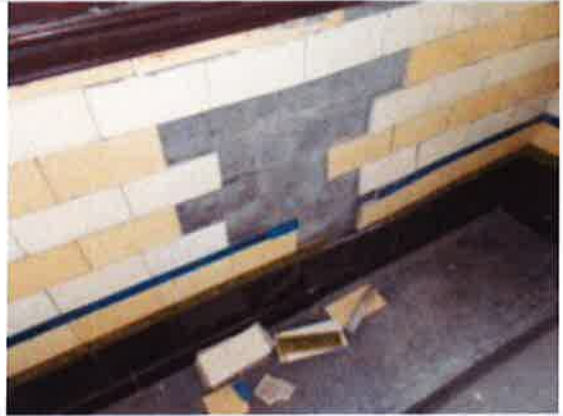
Middle Landing - damaged tiling under window
