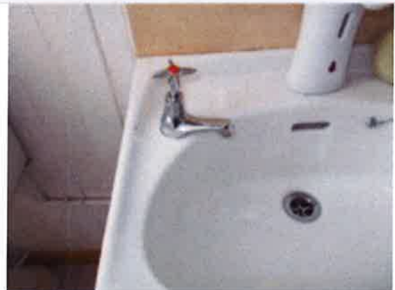
Bathroom - new hot water tap to wash hand basin
