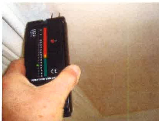
Moisture reading in “green” sector
