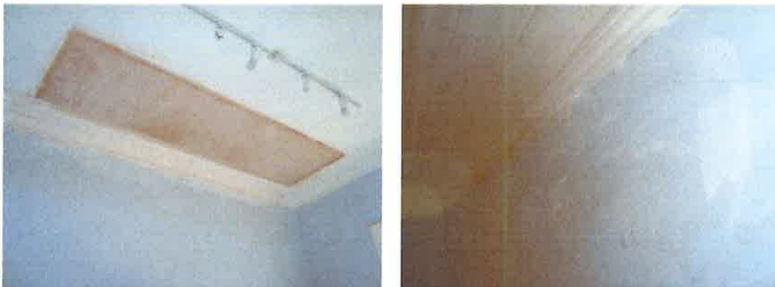
Ceiling /cornice/wall re-plastering
