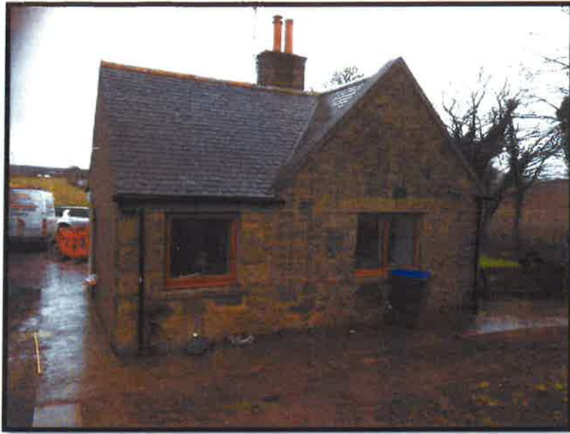
Figure 4 Left gable elevation/side addition - Windows and gutters replaced.
