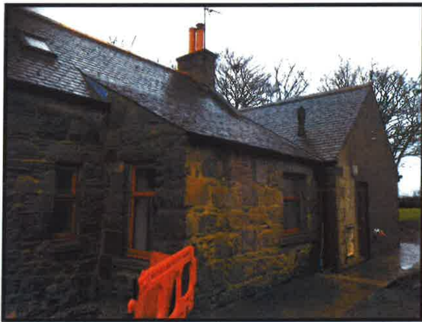
Figure 5 Rear elevation - windows and guttering replaced, new boiler flue present.
