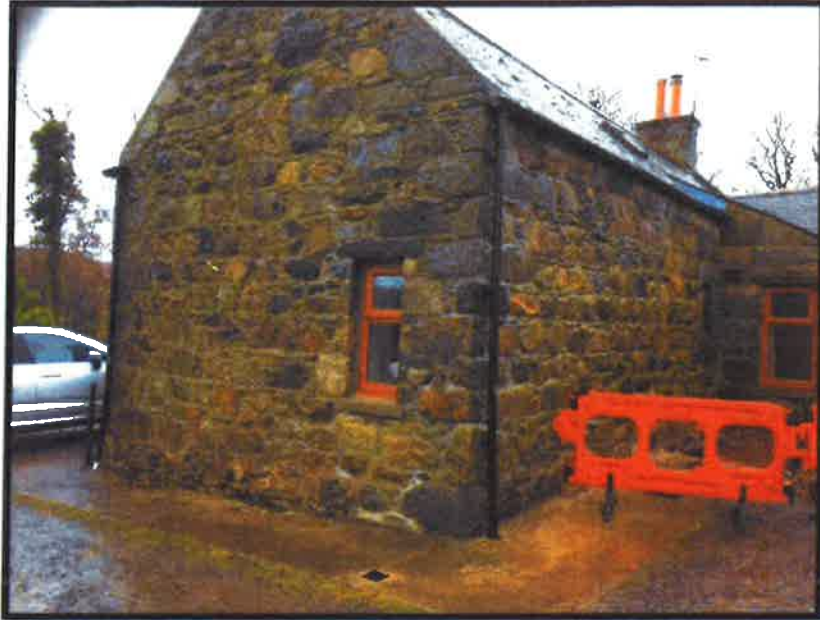
Figure 6 Rear left corner - both cracked areas re-pointed, windows and guttering replaced.
