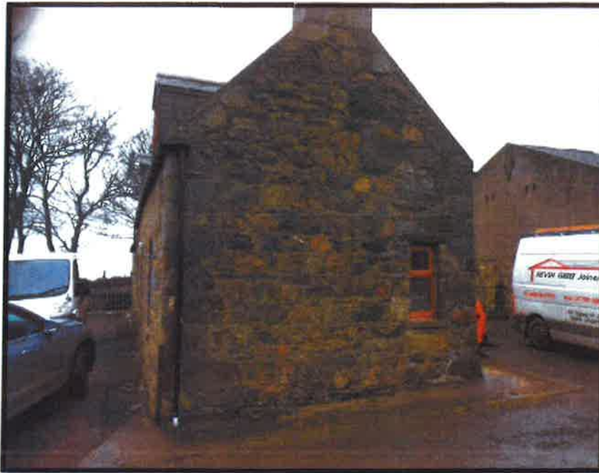
Figure 2 Right hand gable elevation - cracks re-pointed, window replaced.
