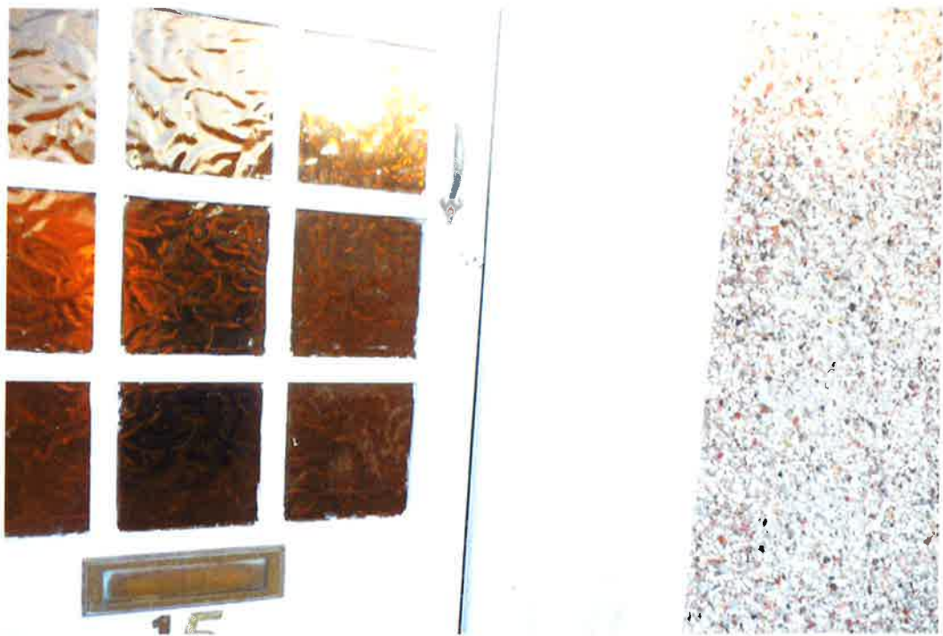
Door detail – see neoprene strip on opening vertical aspect
