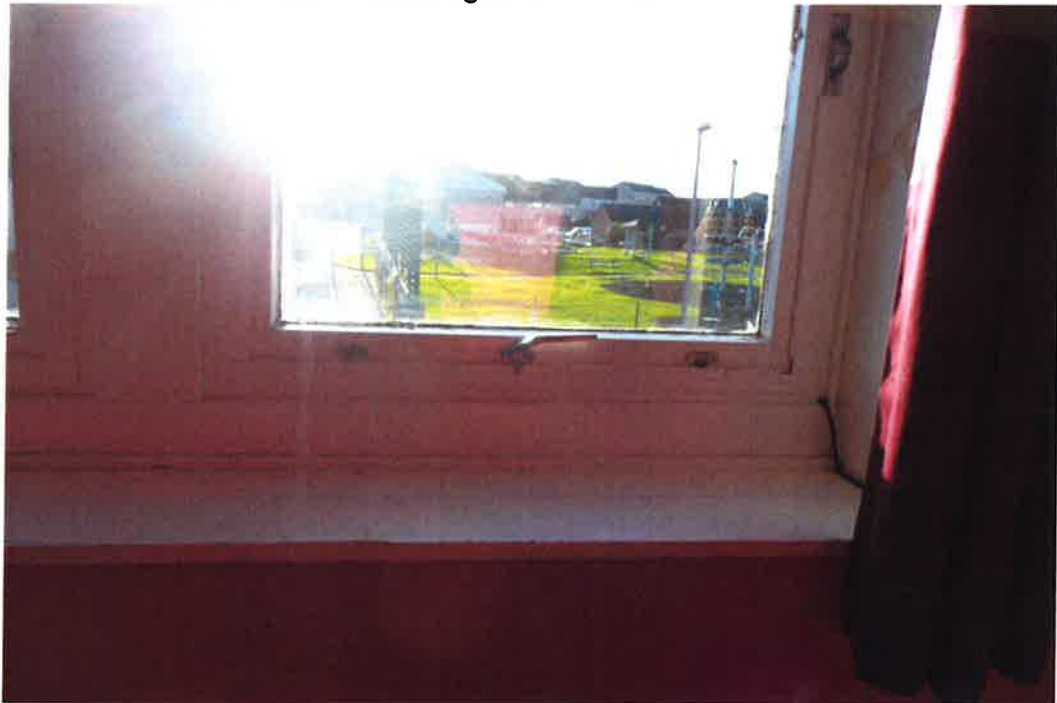
Bedroom window – central locking handle fitted
