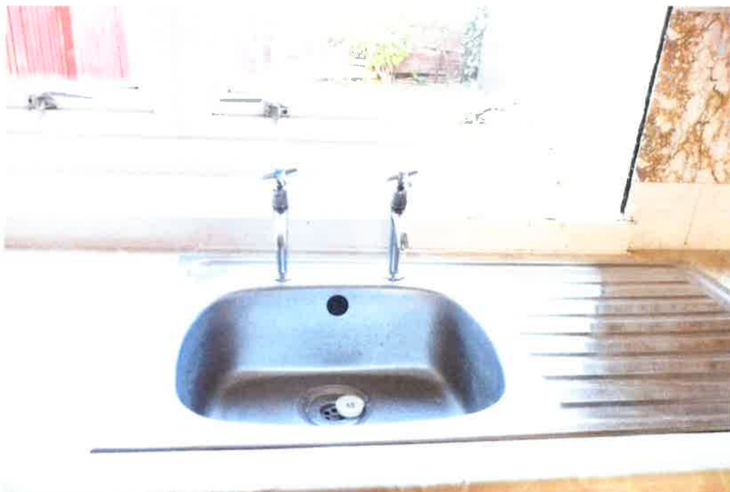
Mastic seal to sink upstand
