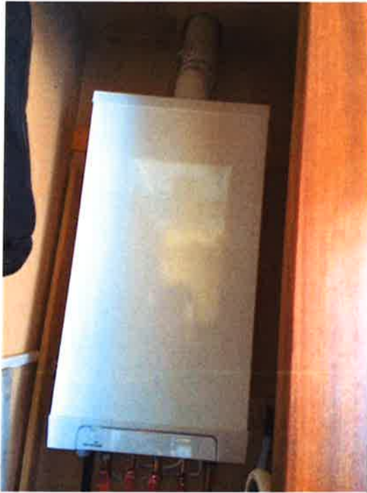
Replacement gas boiler - entrance hall cupboard
