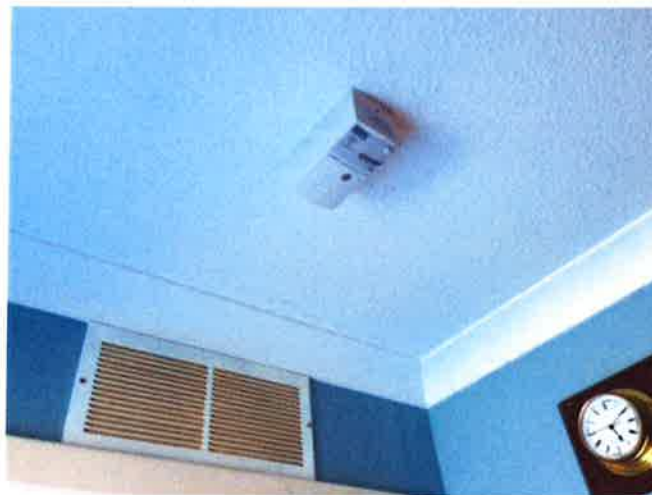
Carbon monoxide detector – entrance hall
