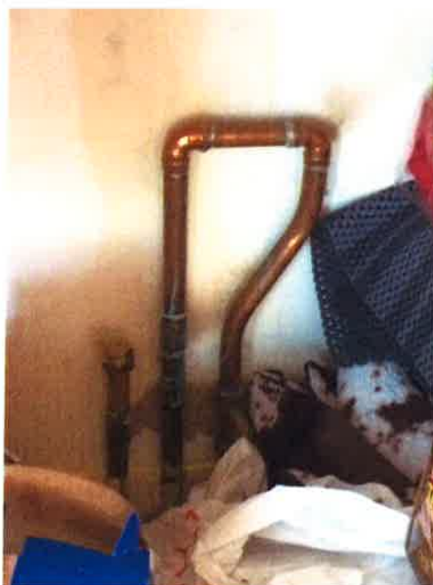
Hot water cylinder tank removed and pipework capped – kitchen cupboard
