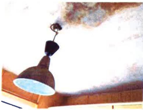
Light fitting in kitchen next to damp patch on ceiling
