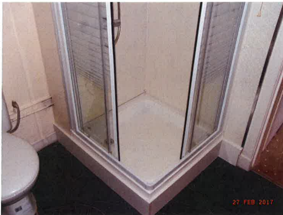
Shower Room (shower unit)
