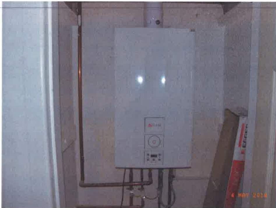
Replacement central heating boiler
