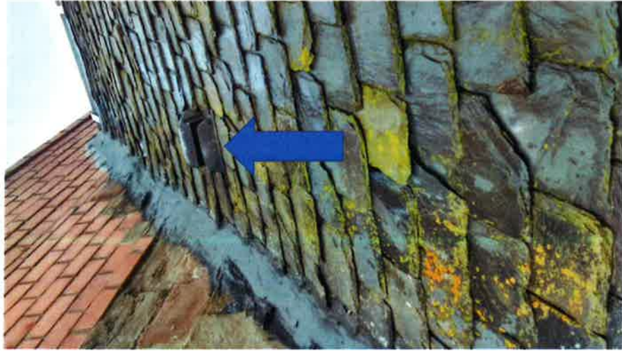
5a) External view of ventilator
