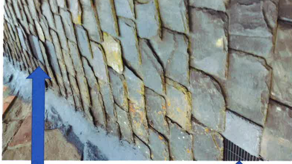
Ventilator removed and replaced with slate ventilation system
