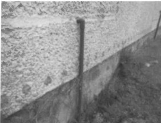
DPC injected to base of external walls
