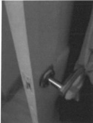
Double bedroom to rear - original door - defective door handle and catch
