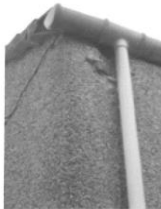
Front elevation - roughcast cracked/spalling/ boss
