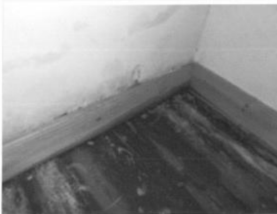
Front double bedroom (left) water damage to walls/skirting and floor adjoining front shower room
