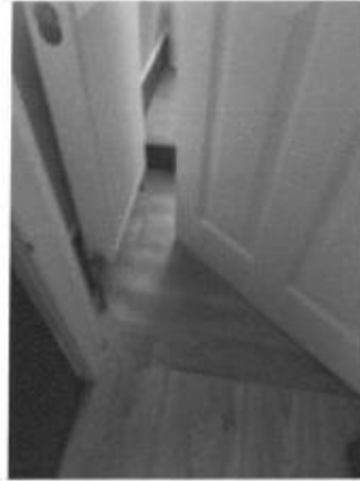
New door to front shower room - door sticking on vinyl floor
