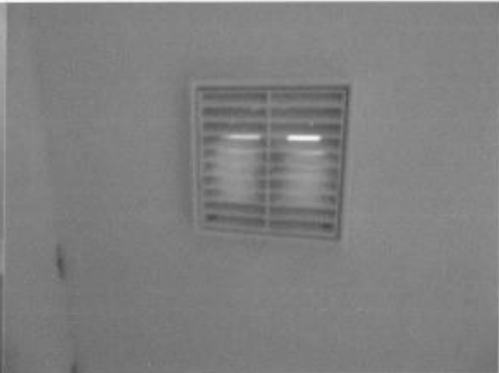
Rear bathroom - vent to external wall
