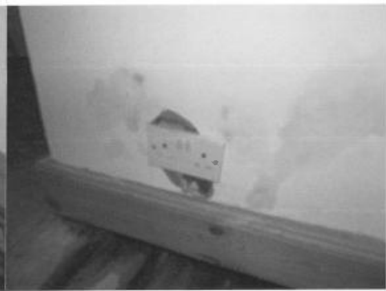
Front double bedroom (left) damage to plasterboard surrounding double socket on wall adjoining front shower room
