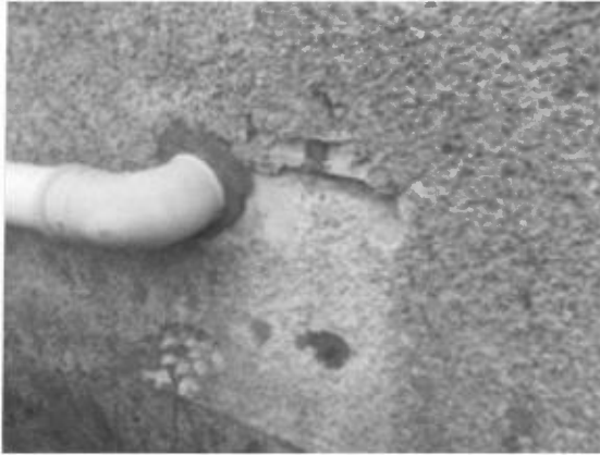
Front elevation - roughcast cracked/spalling/ boss
