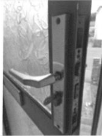
Front door - defective lock/loose handle
