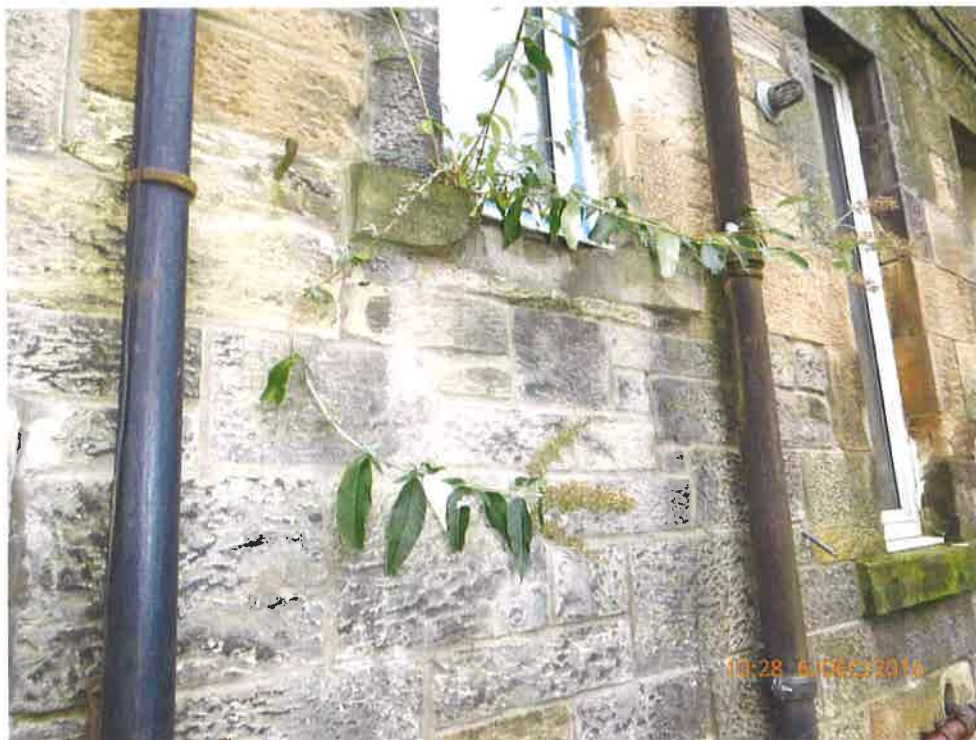
Vegetation growth in bathroom window sill
