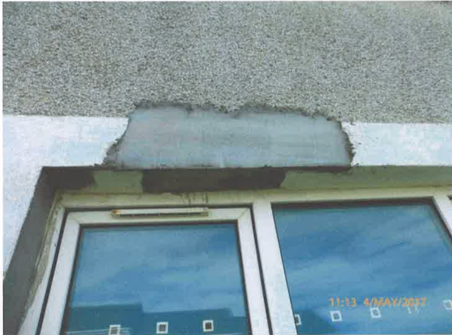
Repair over living-room window
