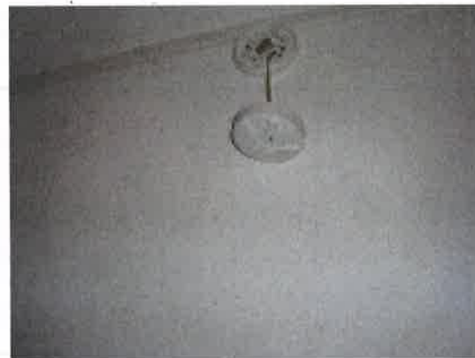
LOOSE FITTING HEAT DETECTOR IN KITCHEN
