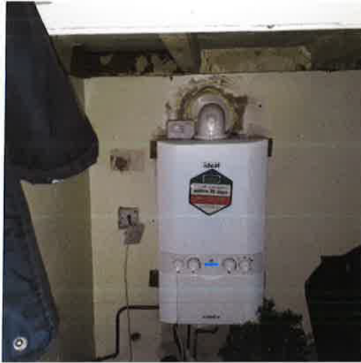
5 Boiler – note CO2 detector on top of boiler unit
