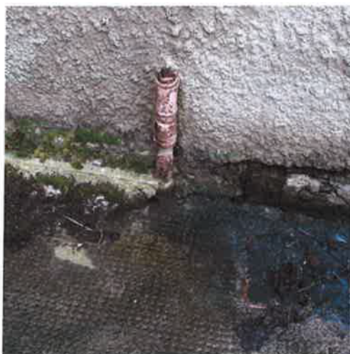
7 Blocked rear external drainage outlet from the washing machine
