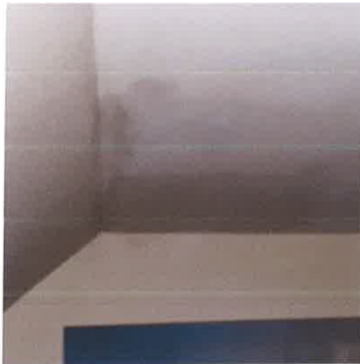
6 Example of internal dampness due to faulty roof slating
