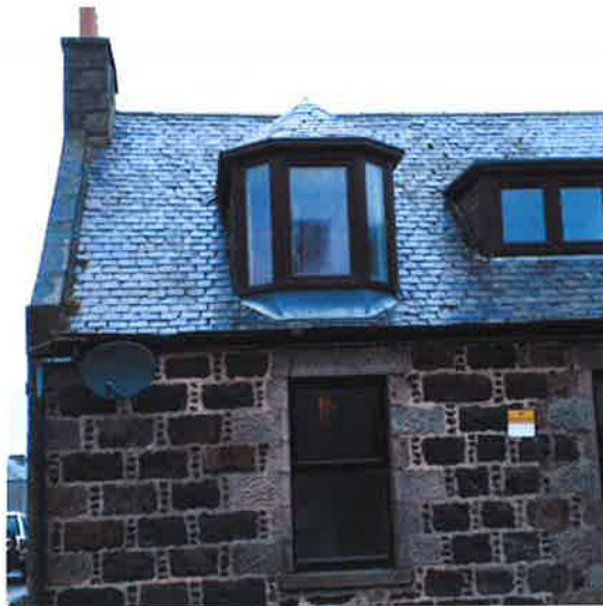
2 Front elevation – slipped and missing slates evident
