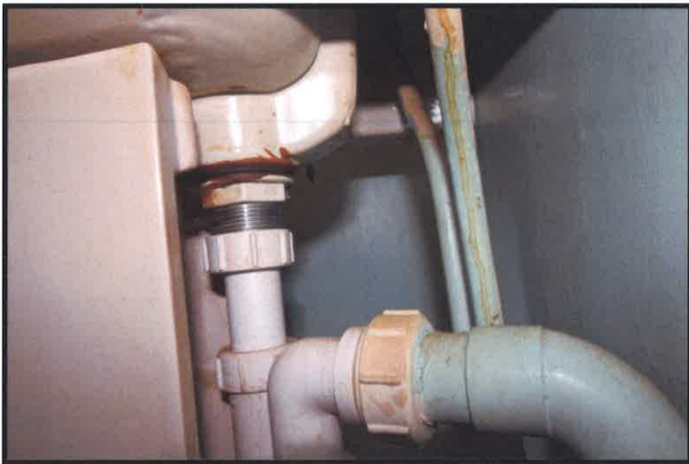
Figure 8 Basin - leak at pipe/basin junction.
