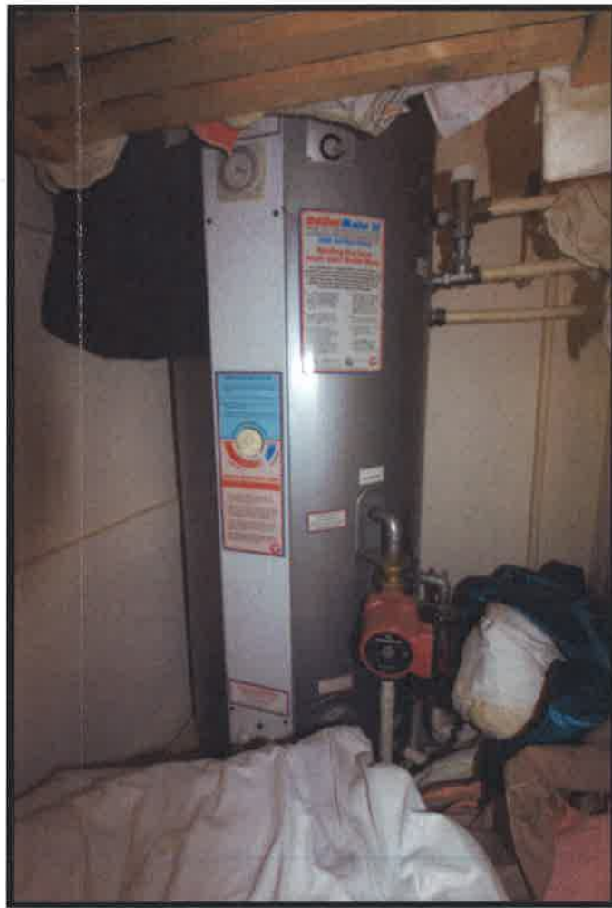
Figure 12 Hot water cylinder.
