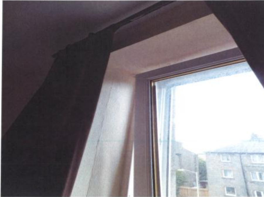
Front bedroom window recess
