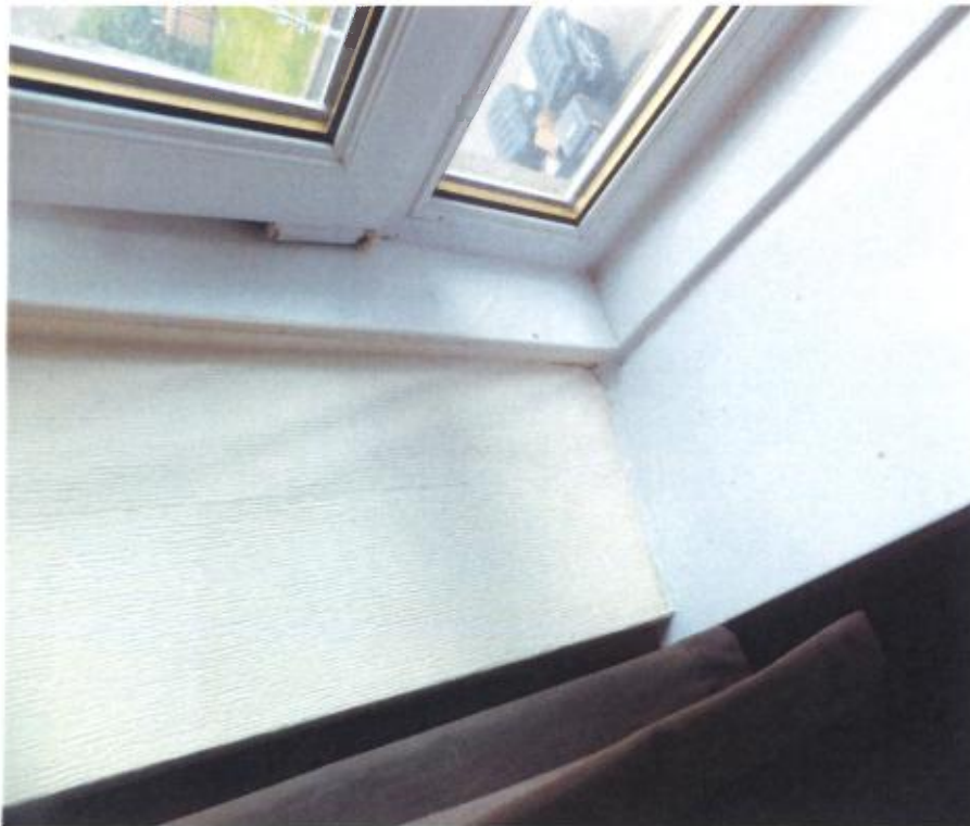
Front bedroom windowsill
