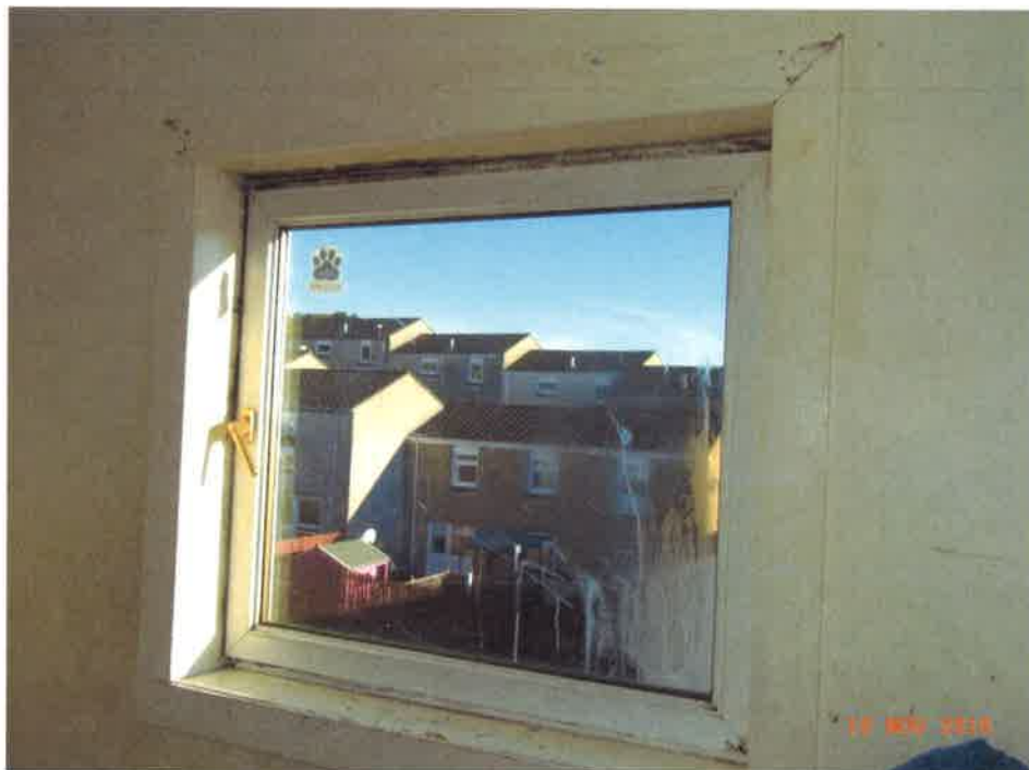
Condensation/mould at Bedroom (4) window
