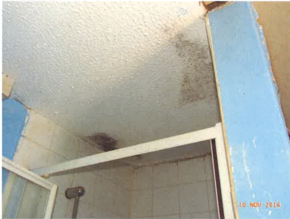
Condensation/mould above shower in Bathroom
