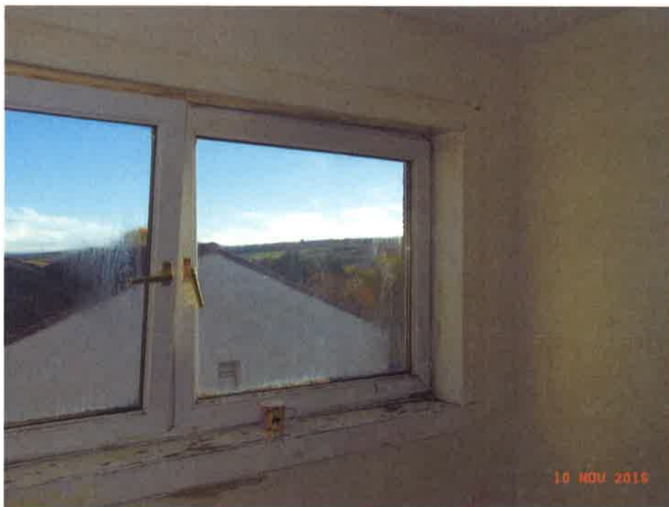
Condensation/mould at Bedroom (3) window
