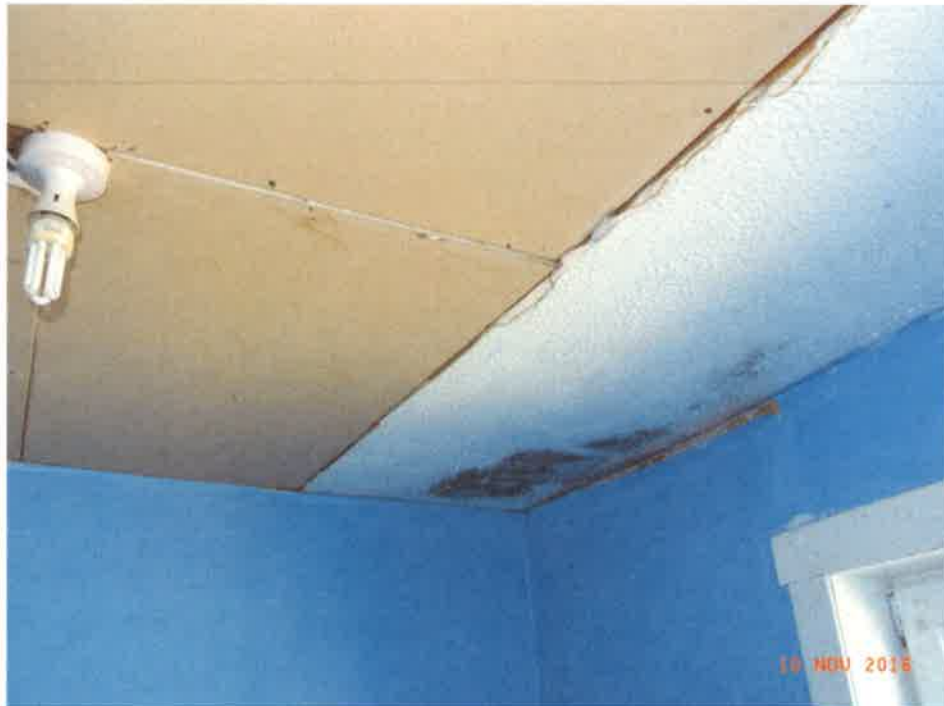
Condensation/mould on Bathroom ceiling
