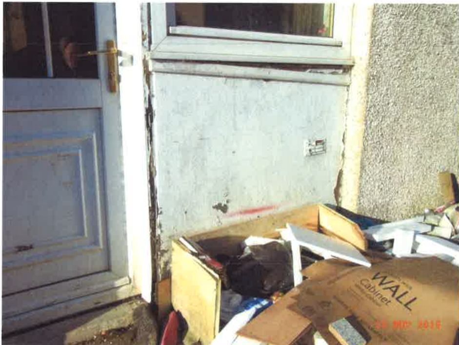
Damaged fascia below kitchen window/adjacent to back door.
