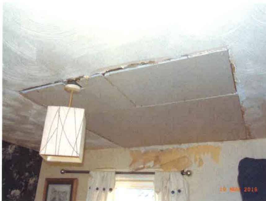
Damage to Living Room ceiling
