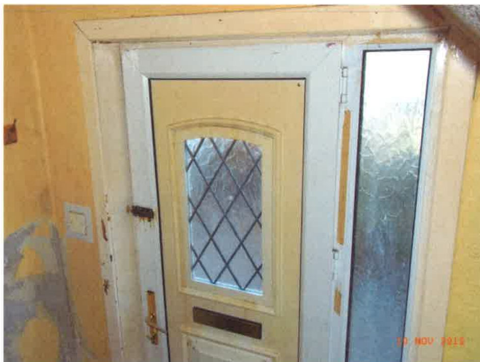
Front door poorly fitting with loose glazing
