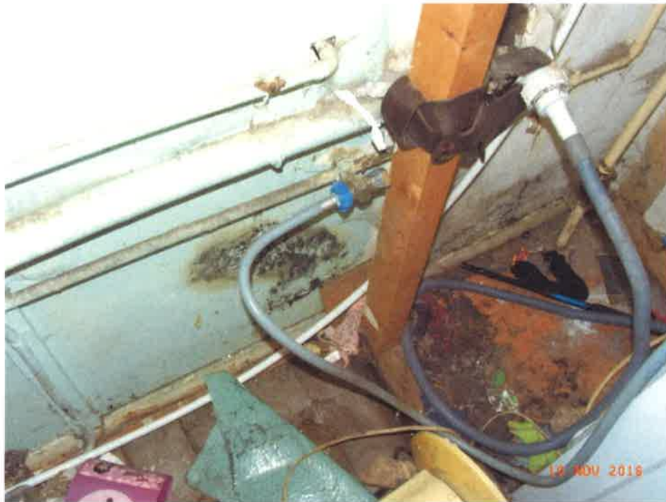
Mould in ground floor cupboard
