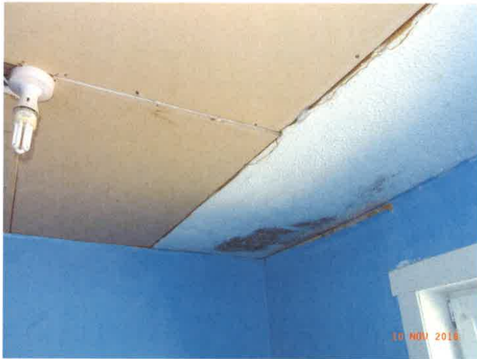
Damage to Bathroom ceiling
