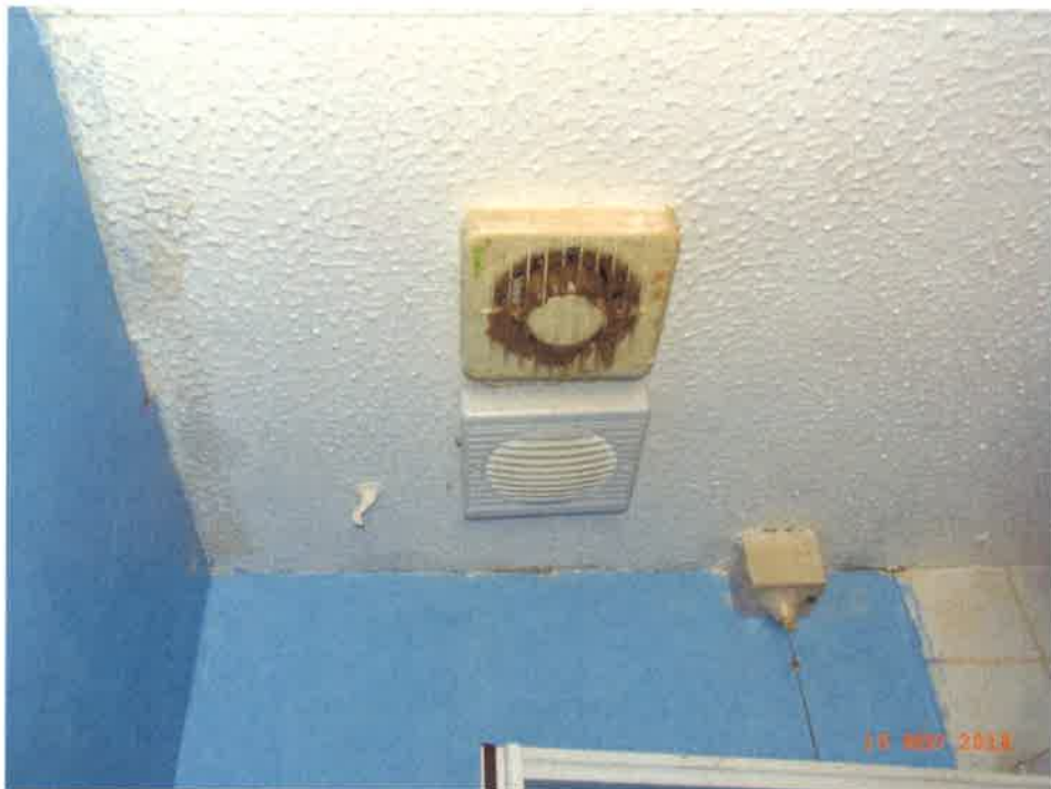
New extractor fan fitted in Bathroom
