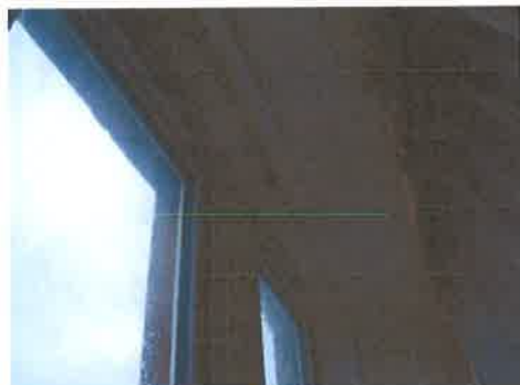
5. WATER LEAKS AT FRONT ROOM WINDOW LINTOL:
