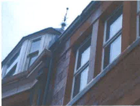
7. WATER LEAKING AT DEFECTIVE FRONT GUTTER
