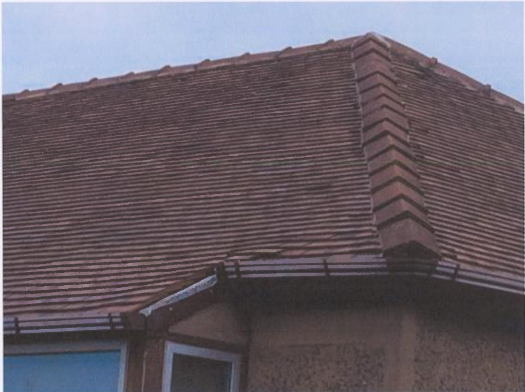
Roof – front pitch – 10 February 2017
