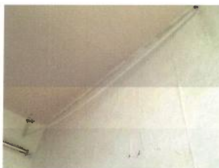
13 September 2017 Hanging PVC conduit wiring
