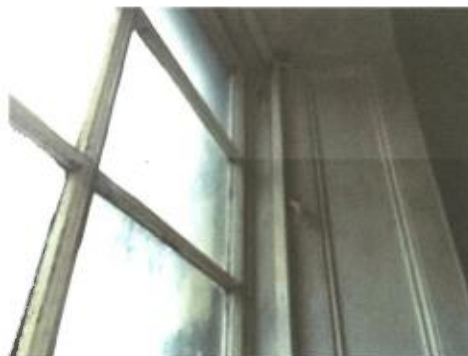
13 September 2017 Missing sash cord kitchen window
