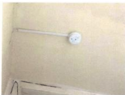
13 September 2017 Kitchen heat detector
