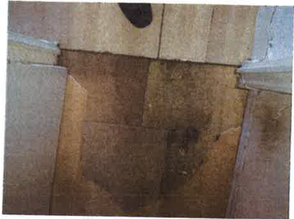
8 Defective vinyl flooring within Kitchen.
