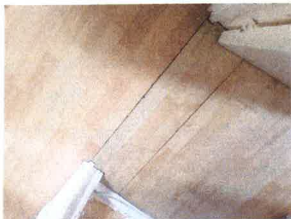
20 Loose laminate at threshold.
