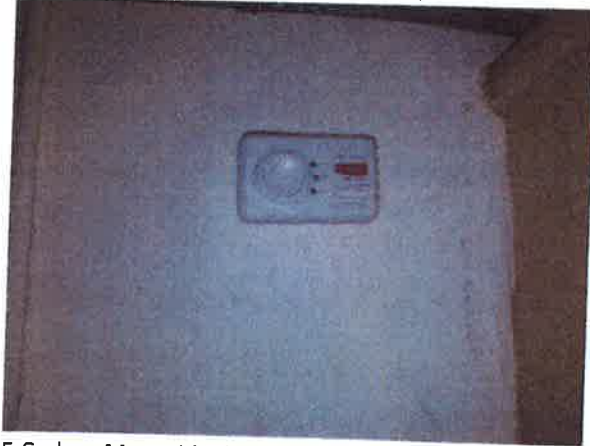
5 Carbon Monoxide detector present within Kitchen.
