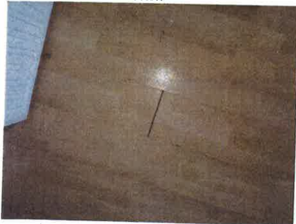
11 Further example of open joint to laminate floor.
