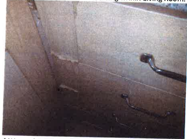
4 Water damage to kitchen drawer units.
