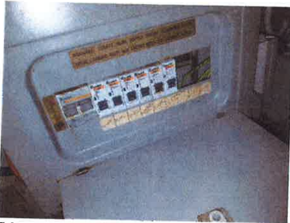
7 Consumer Unit – open to wiring.
