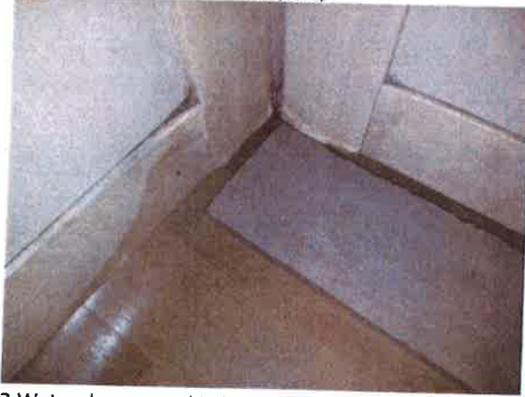
3 Water damage to kitchen base units.
