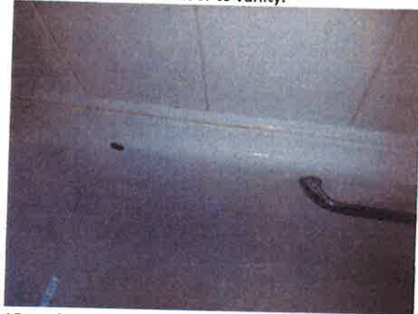
15 Further minor damage to enamel and seals intact.
