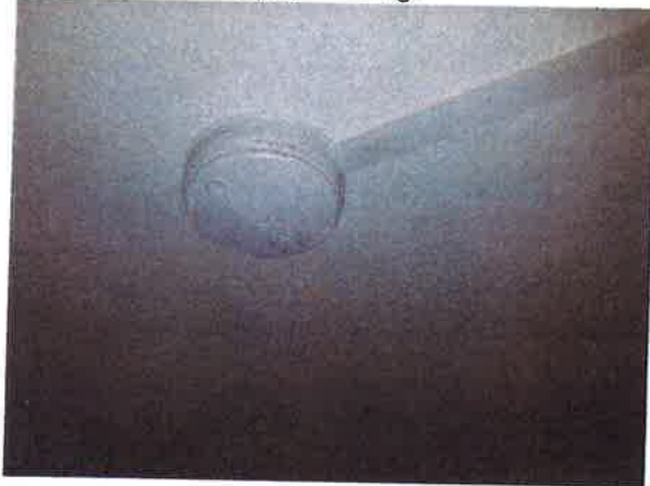
9 Hardwired smoke detector.
