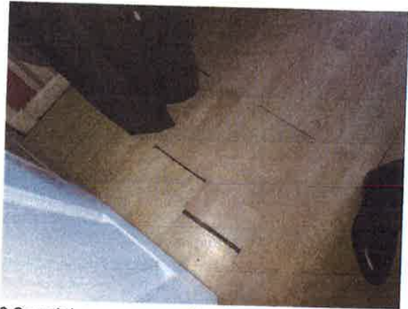
2 Open joints to laminate flooring within Living Room.
