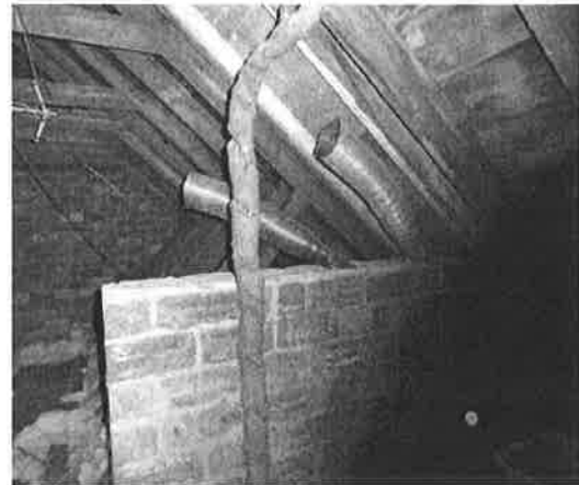
4. Remains of chimney breast in attic
