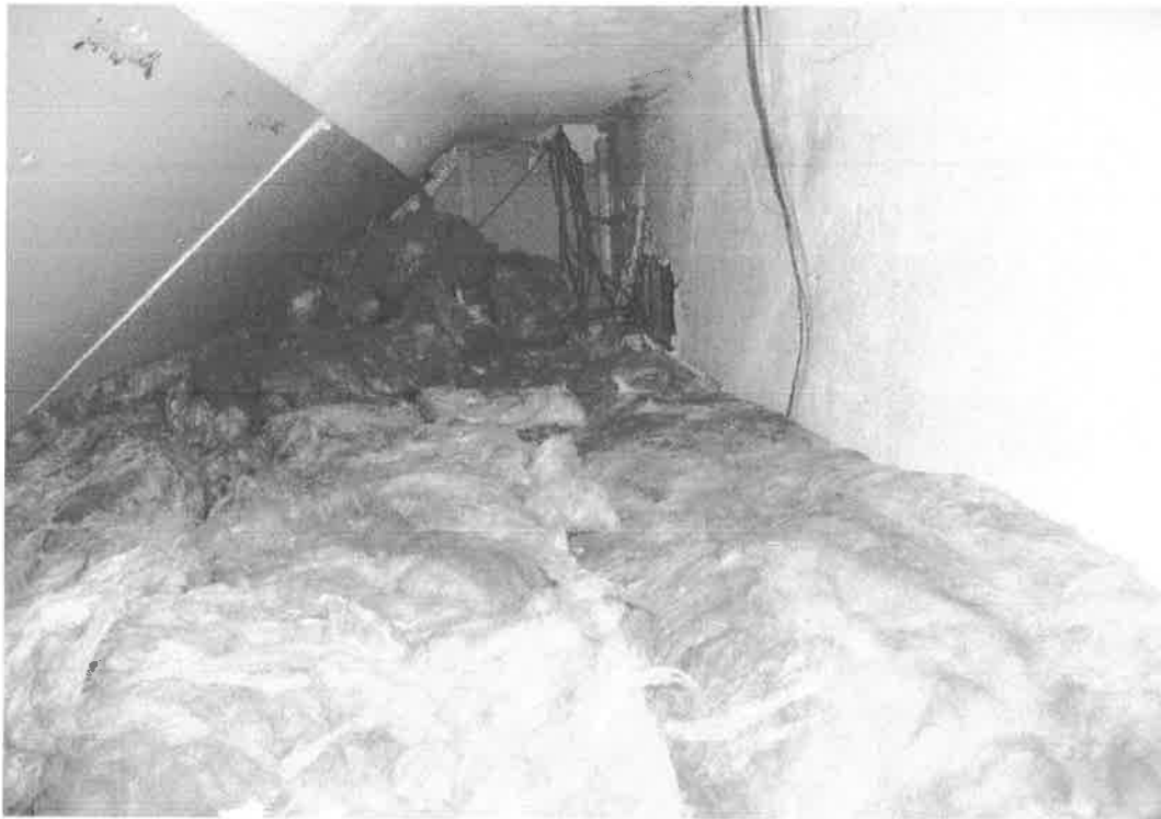
Insulation of space above entrance corridor
