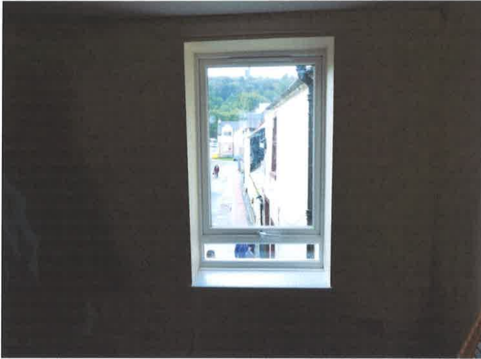
Bedroom window – replacement UPVC unit
