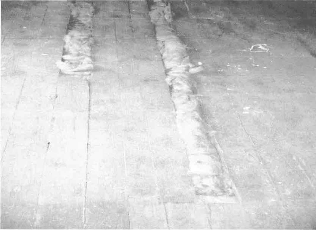
Insulation of loft showing glass quilt forced into gaps between boards
