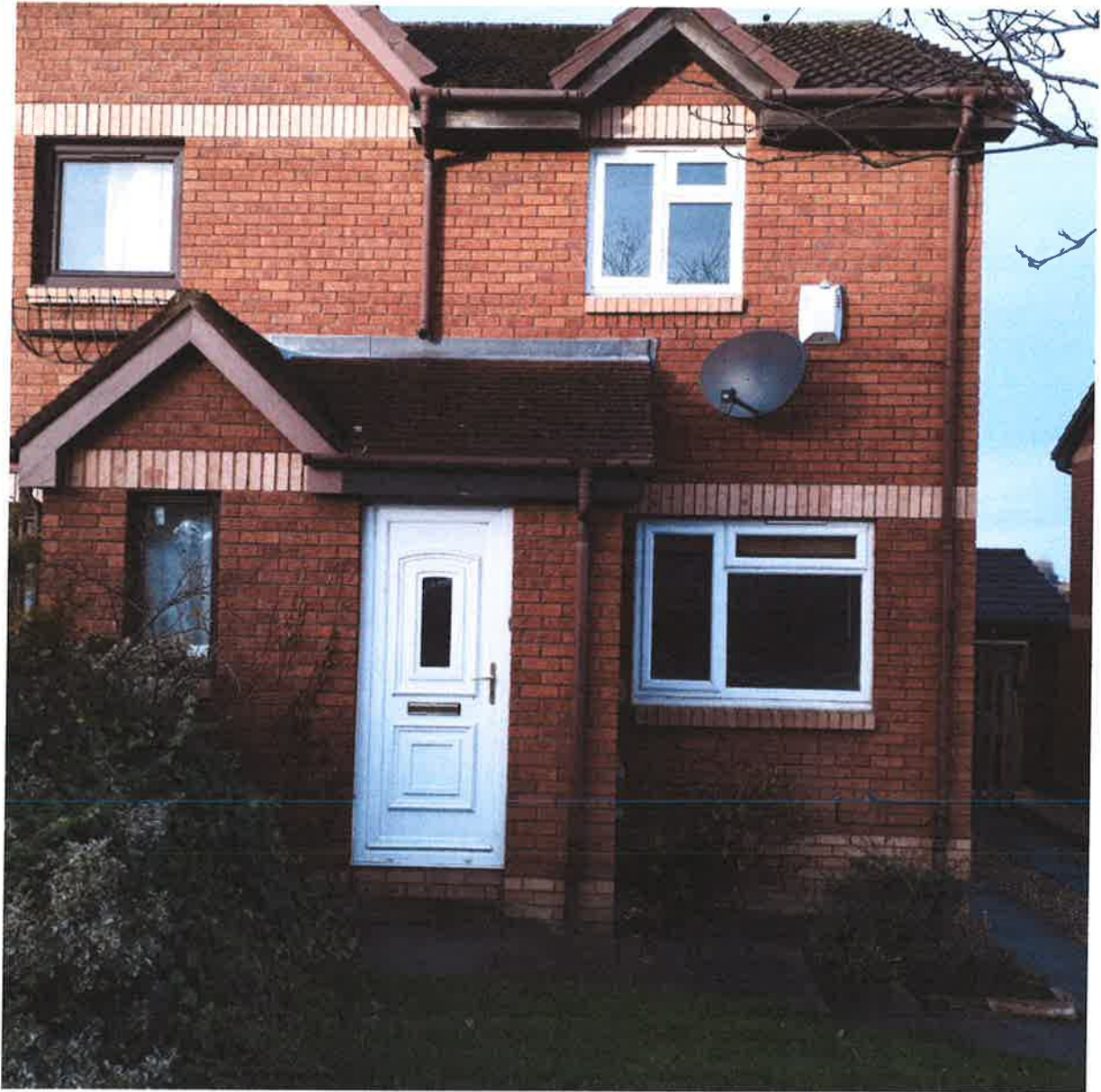
1 Front elevation of 183 Upper Craighour
