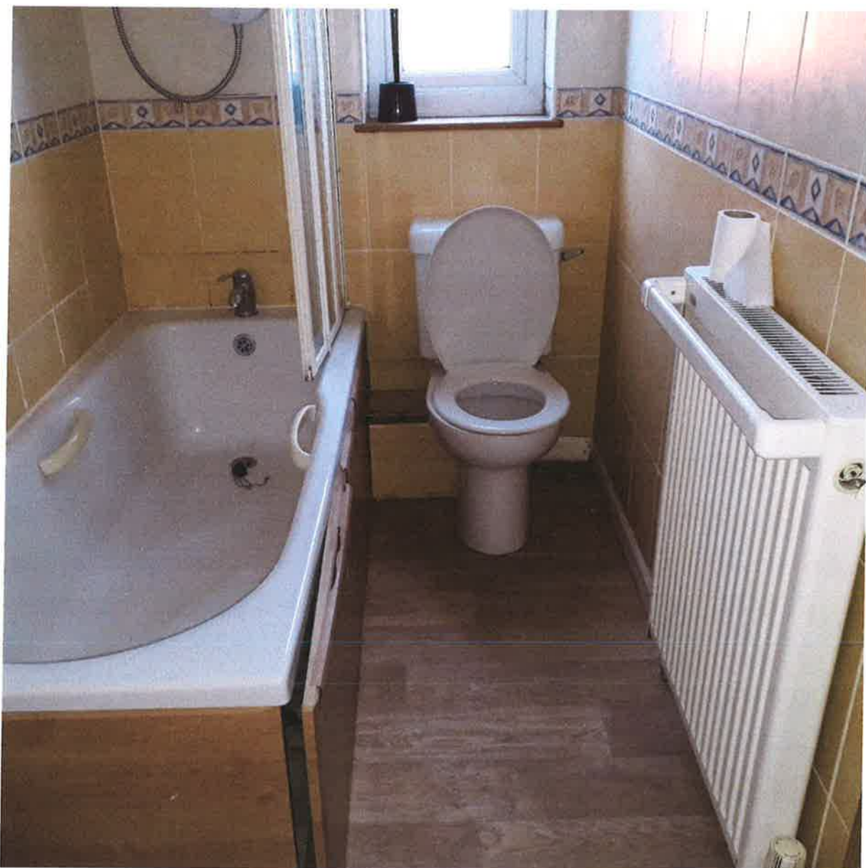
6 View of the recently repaired WC.
