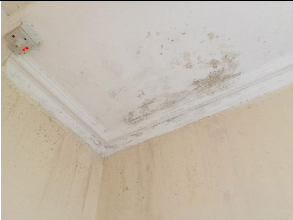
Condensation in the shower room
