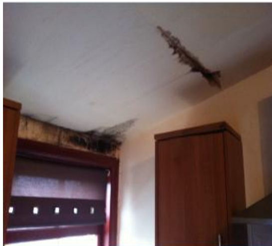
Mould within property at time of inspection
