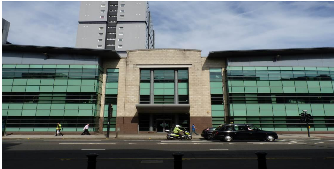
Prhp and hohp offices at Europa Building, Argyle Street, Glasgow
