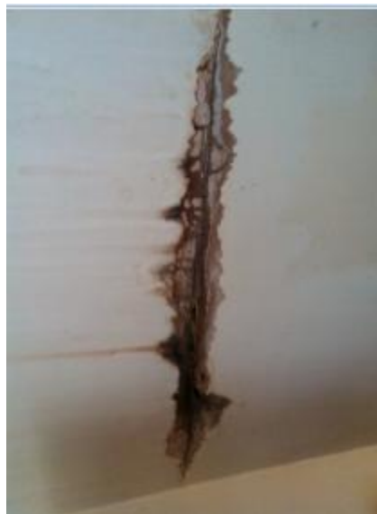
Crack on ceiling caused by water damage
