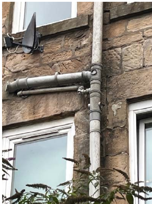
Detail of drainage
