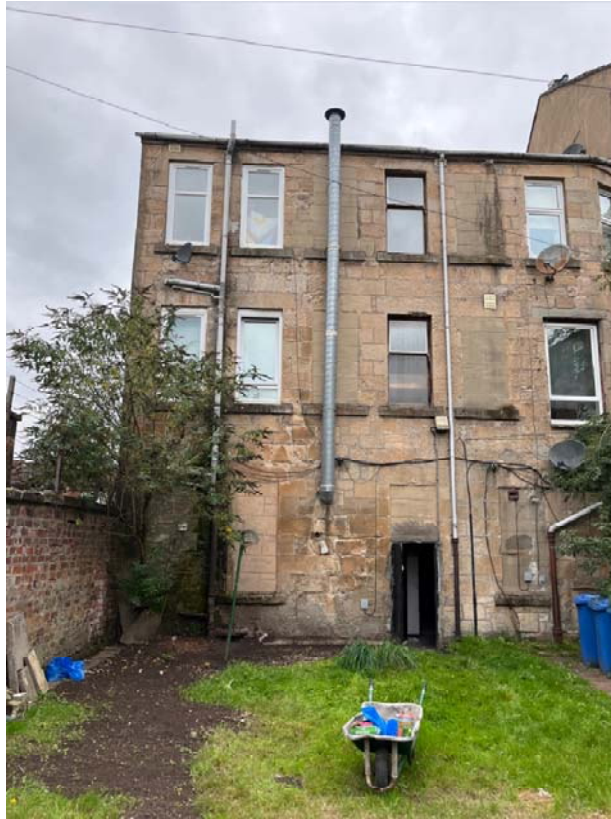
Rear of the building
