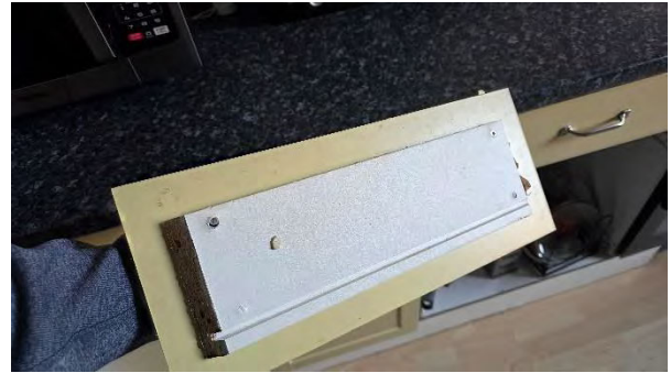
10 Example of retained, failed drawer front
