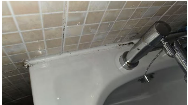
19 Bath installation abutting wall tiling.
