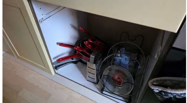
8 Further missing door front to base unit.
