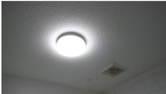
Photo 2 – New appropriate Bathroom light fitting
