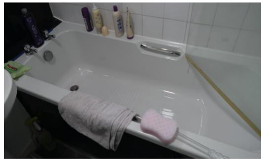
Photo 3 – New bath unit and silicon sealant
