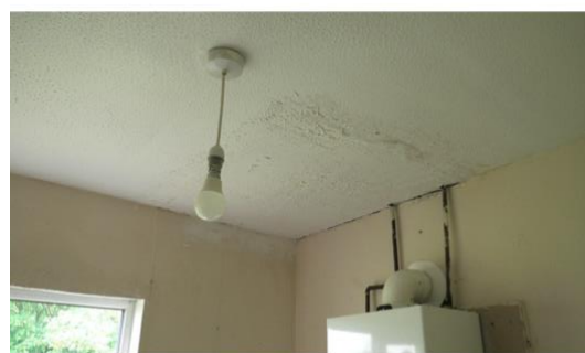
Photo 9 – Dry ceiling above boiler now repaired
