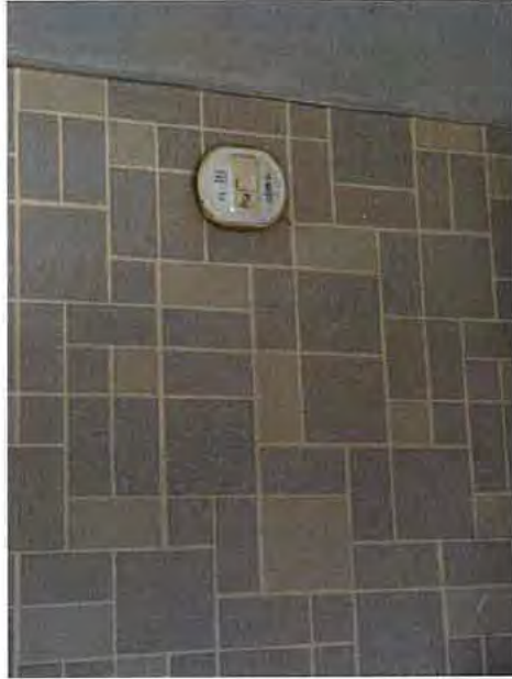
Photograph 9: Landing: Smoke detector – interlinked and in working order
