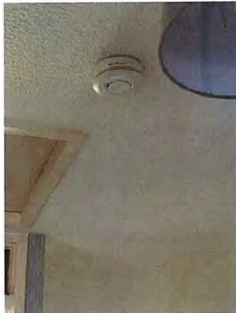
Photograph 9: Landing: Smoke detector – interlinked and in working order
