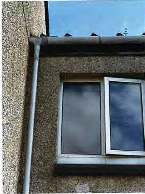
Photograph 28: Section of front guttering
