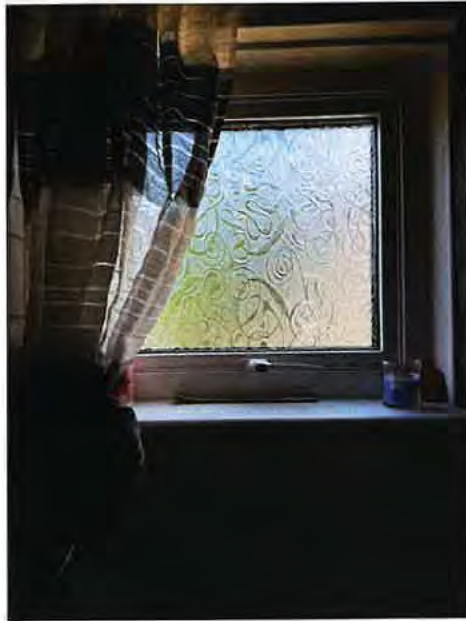
Photograph 4: Downstairs WC: Casement window
