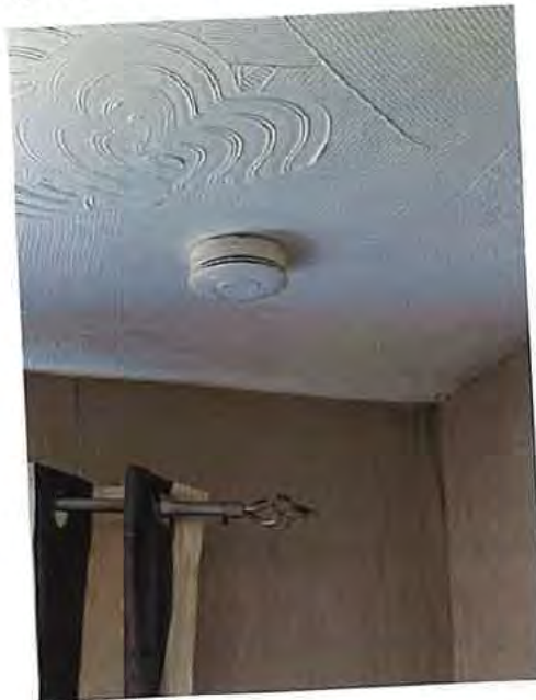
Photograph 3: Living room: Smoke detector - interlinked and in working order
