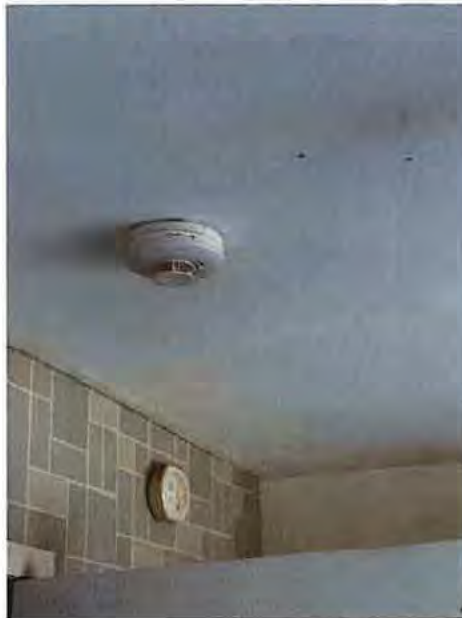
Photograph 7: Kitchen: Heat detector – interlinked and in working order
