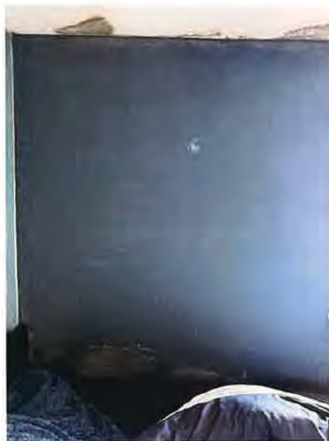
Photograph 13: Bedroom 3: Section of rear wall showing staining and black mould at ceiling level
