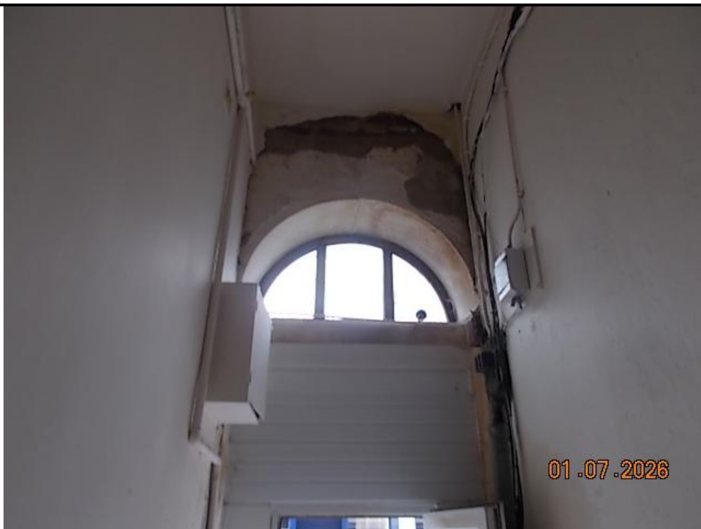
12. Common stairwell above front entrance
