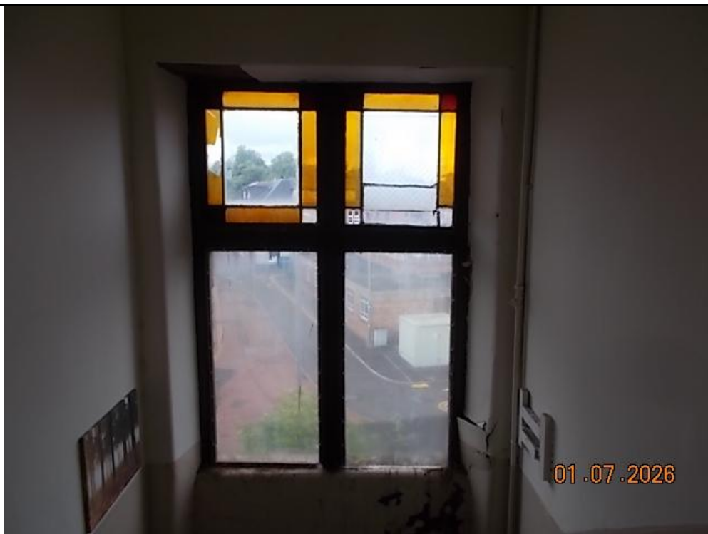
8. Common stairwell at top level
