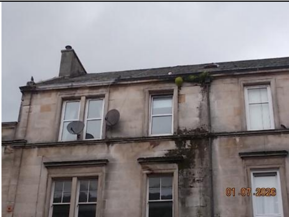
2. Front roof over and elevation of the property
