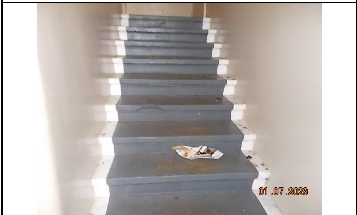
10. Common stairwell leading up to first floor level
