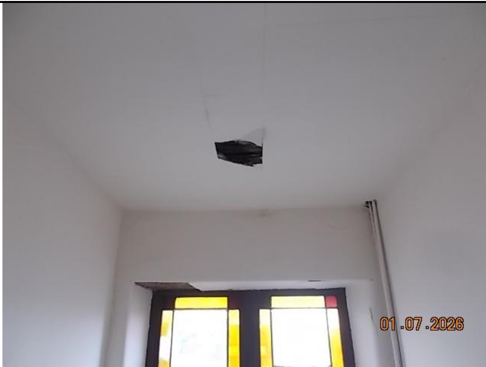
7. Common stairwell at top level
