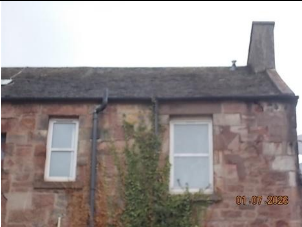
5. Rear roof over and elevation of the property
