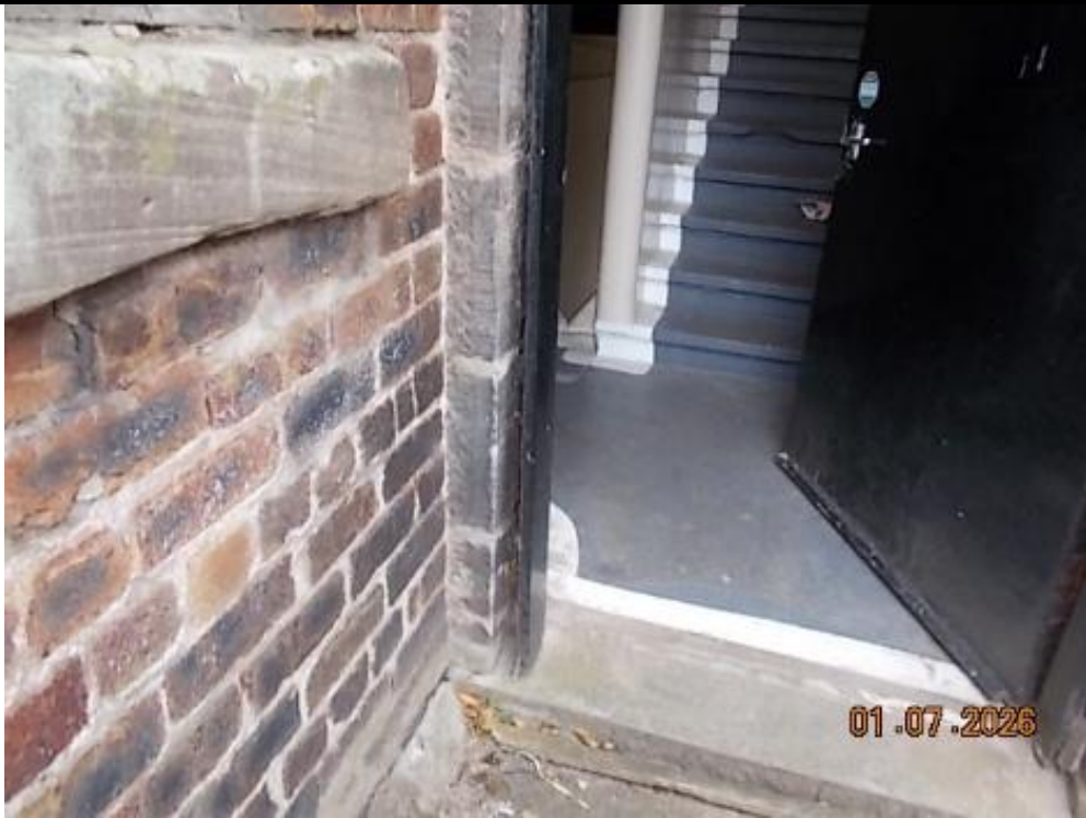
13. Common stairwell rear entrance
