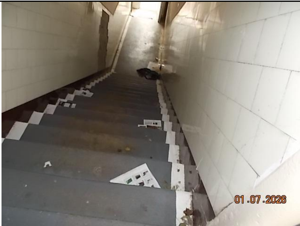
11. Common stairwell leading down to front entrance
