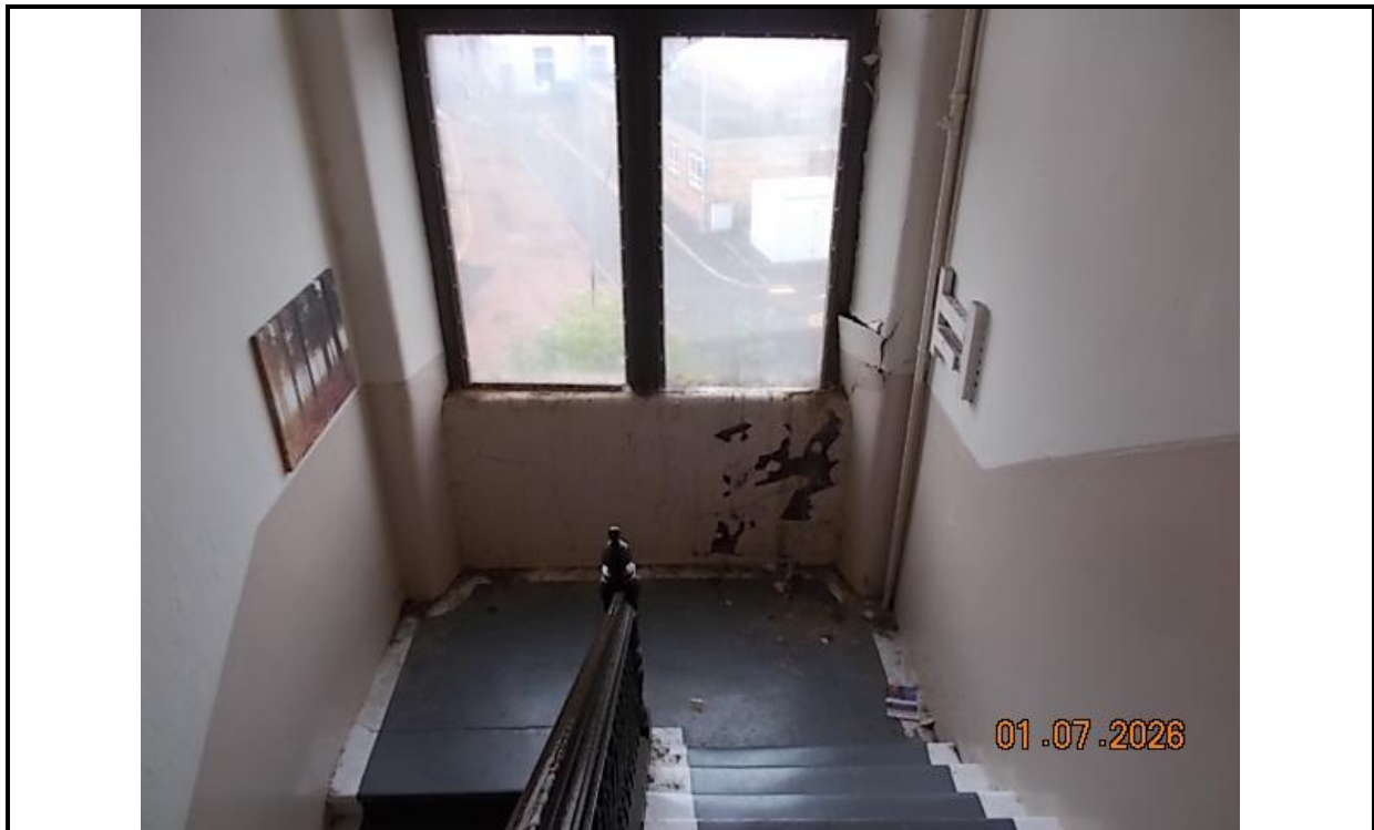
9. Common stairwell at top level
