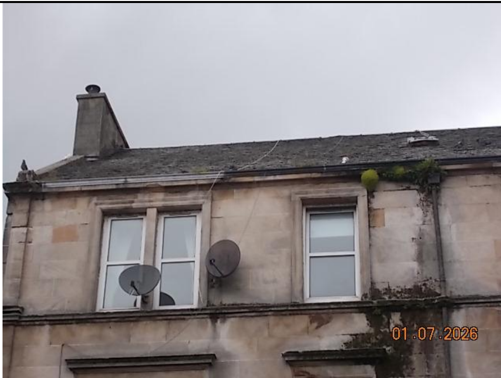
3. Front roof over and elevation of the property
