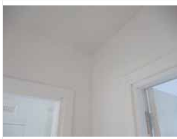
Hall - view of walls/ceiling above kitchen and bathroom door frames
