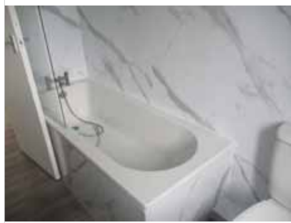
Bathroom - new bath, shower and screen
