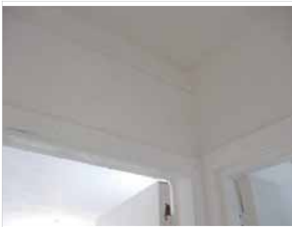
Hall - view of walls/ceiling above kitchen and living room door frames
