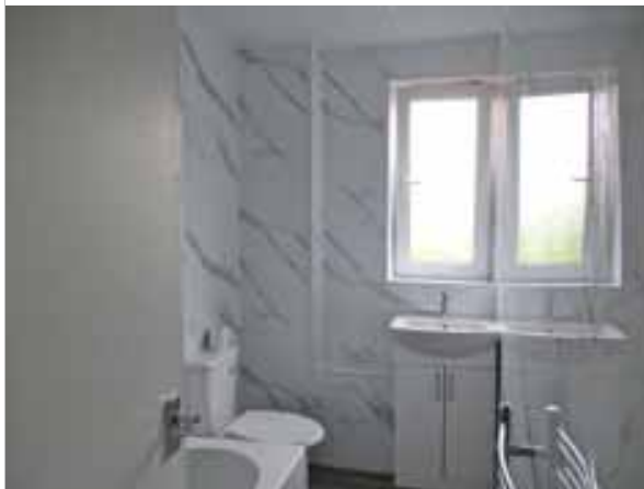
Bathroom - new 3 piece white suite and wet wall cladding
