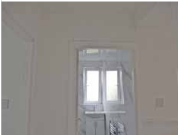
Hall - wall replaced/bathroom door standard renewed
