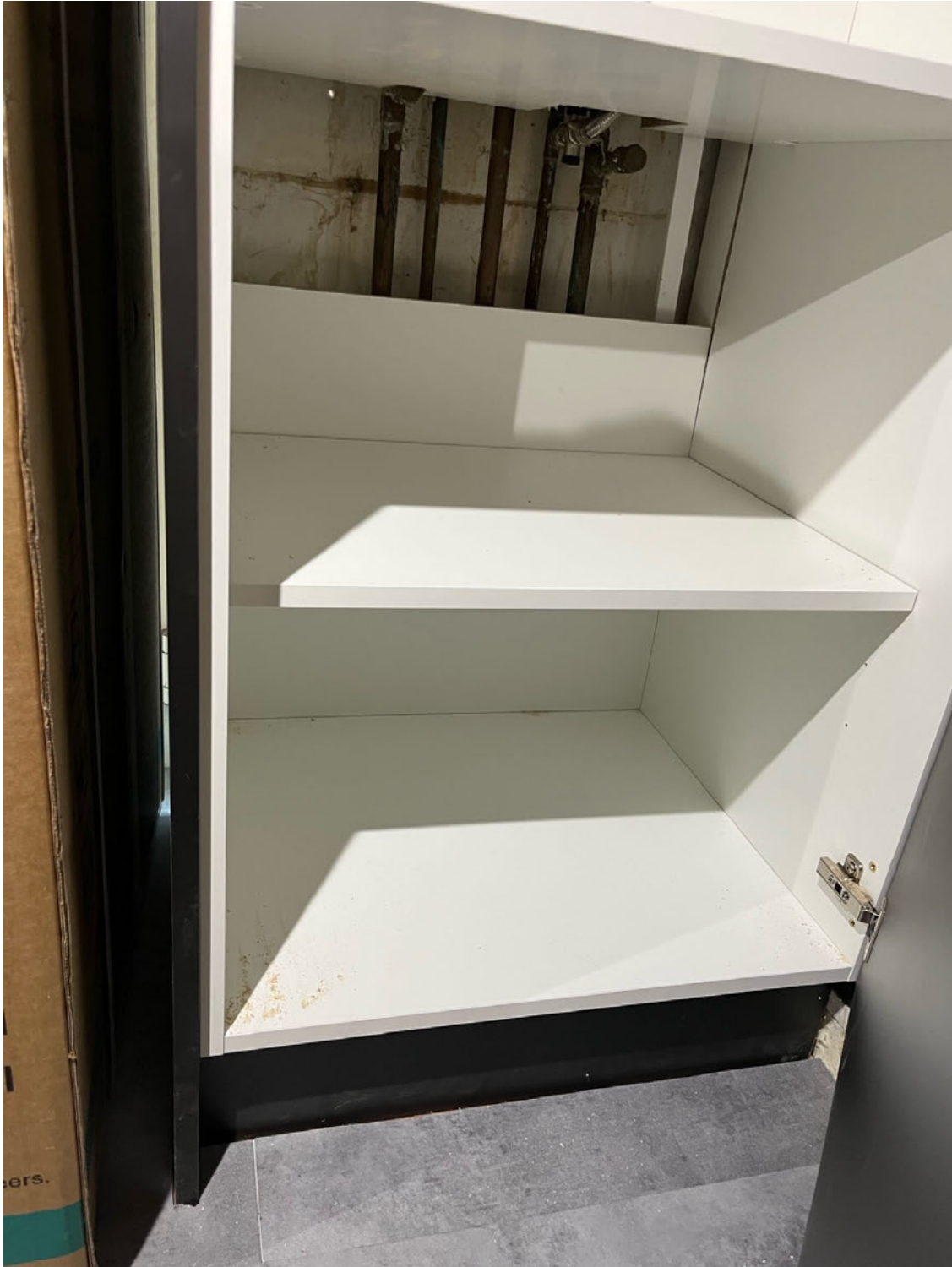
Base below the boiler
