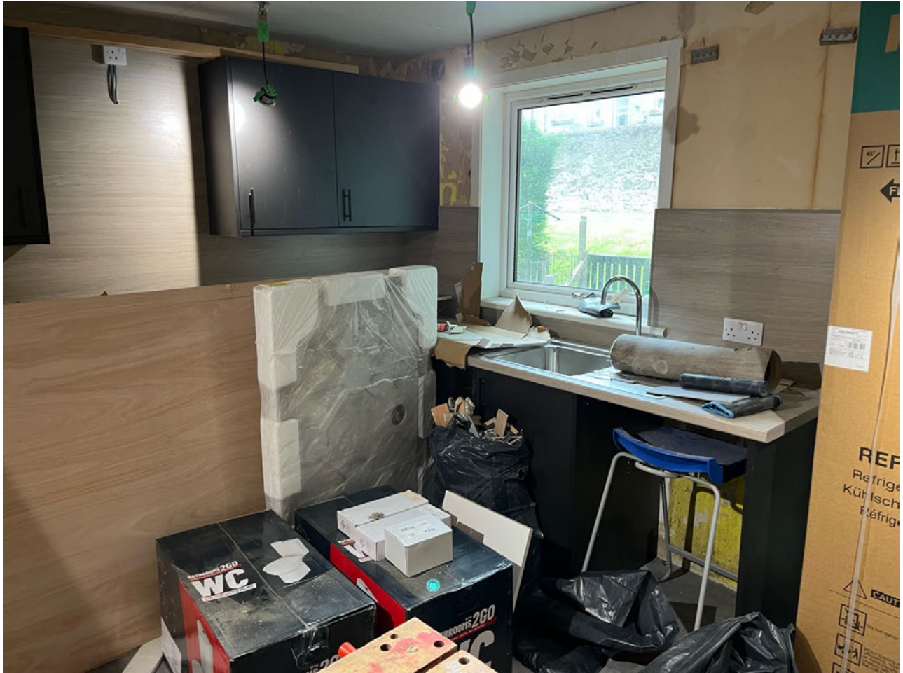
Indication of works being carried out
