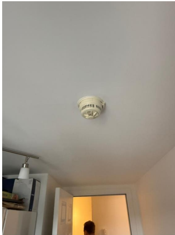
Photograph 15: Hallway: Smoke detector
