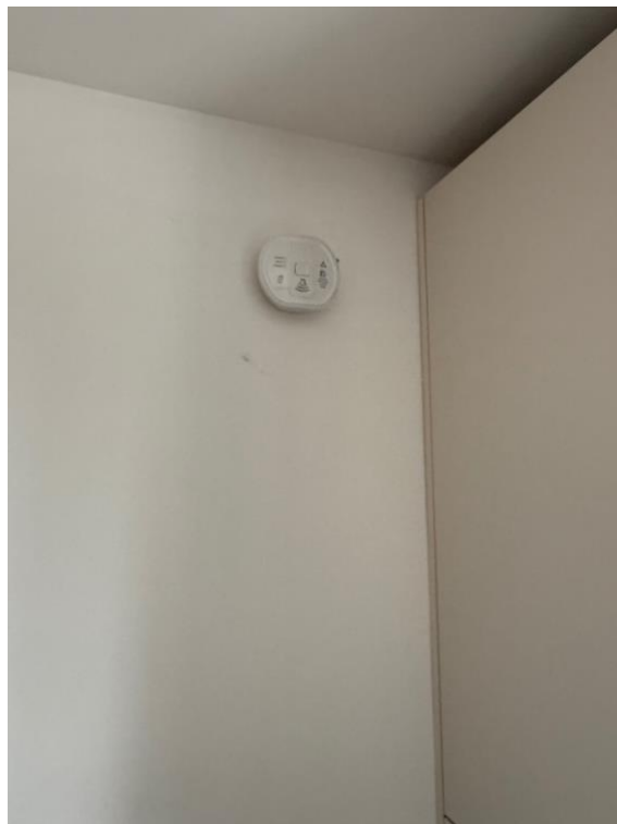
Photograph 13: Kitchen: Carbon monoxide detector
