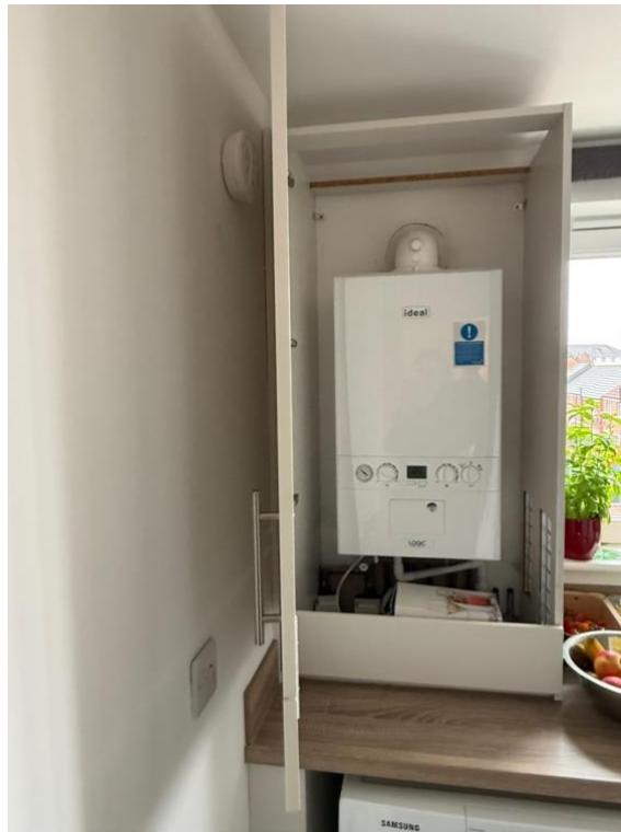
Photograph 13: Kitchen: Carbon monoxide detector
