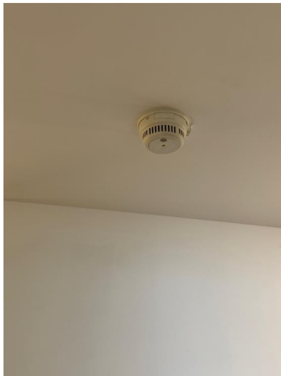
Photograph 15: Hallway: Smoke detector
