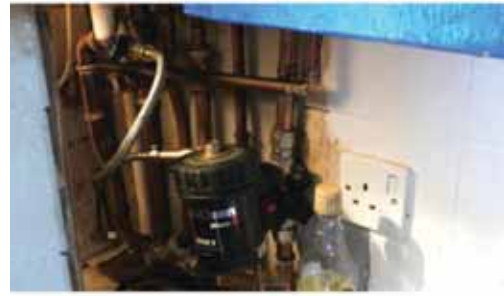
Photo 25 – Boiler pipework revealed
