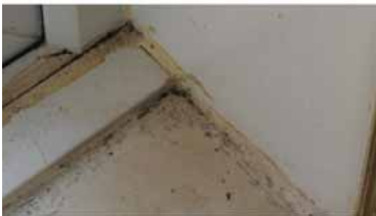
Photo 14 – Mould around living room window
