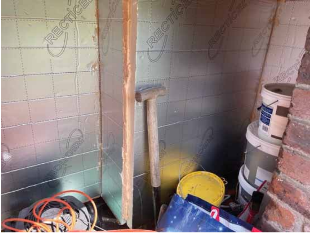
Insulation in outside store
