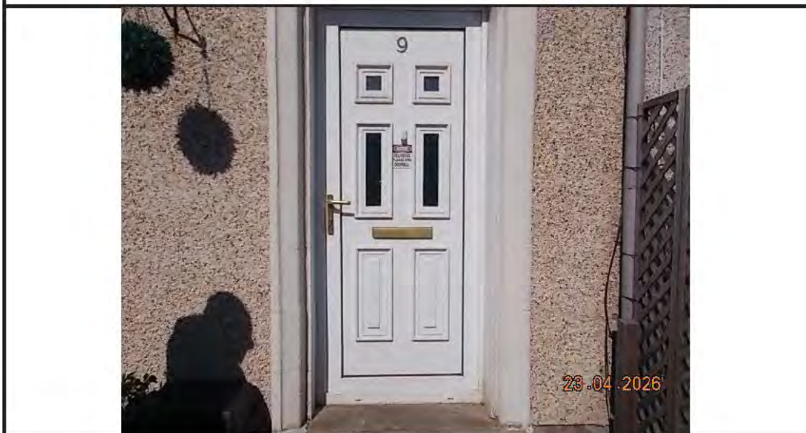
16. Front door outer face (undamaged)
