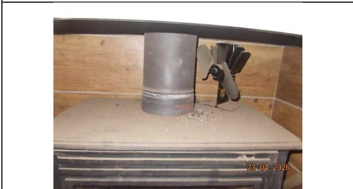
6. Wood burner flue connector
