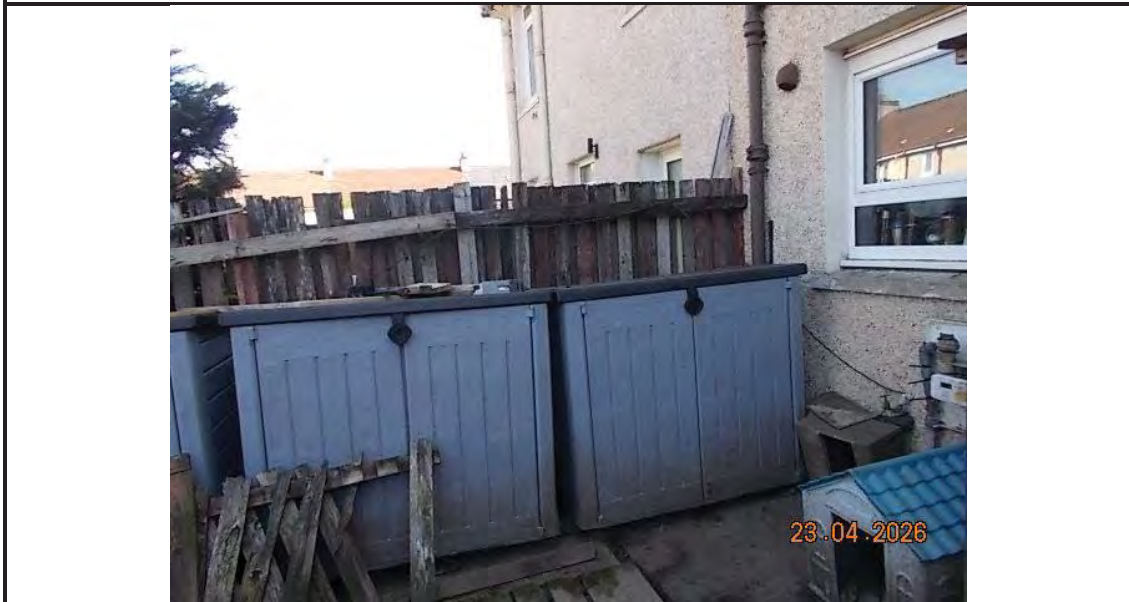
26. Fence to rear of House
