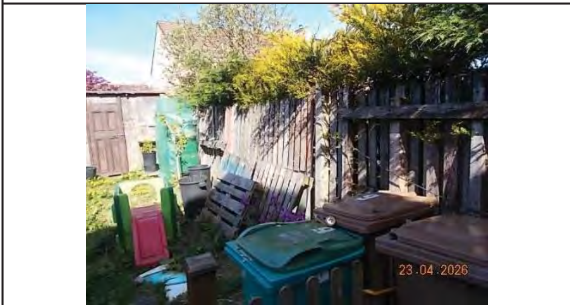
28. Fence to rear of House
