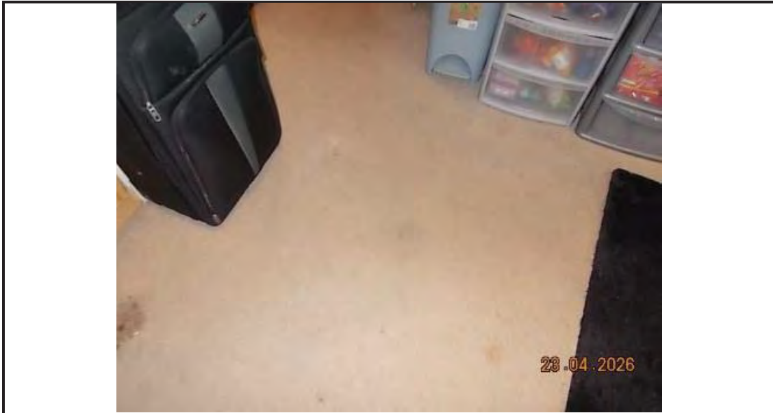
43. Carpet to larger room, first floor at front of property
