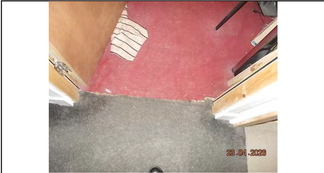
41. "Cover strip" missing at carpet joint, smaller room, first floor at front of property to landing
