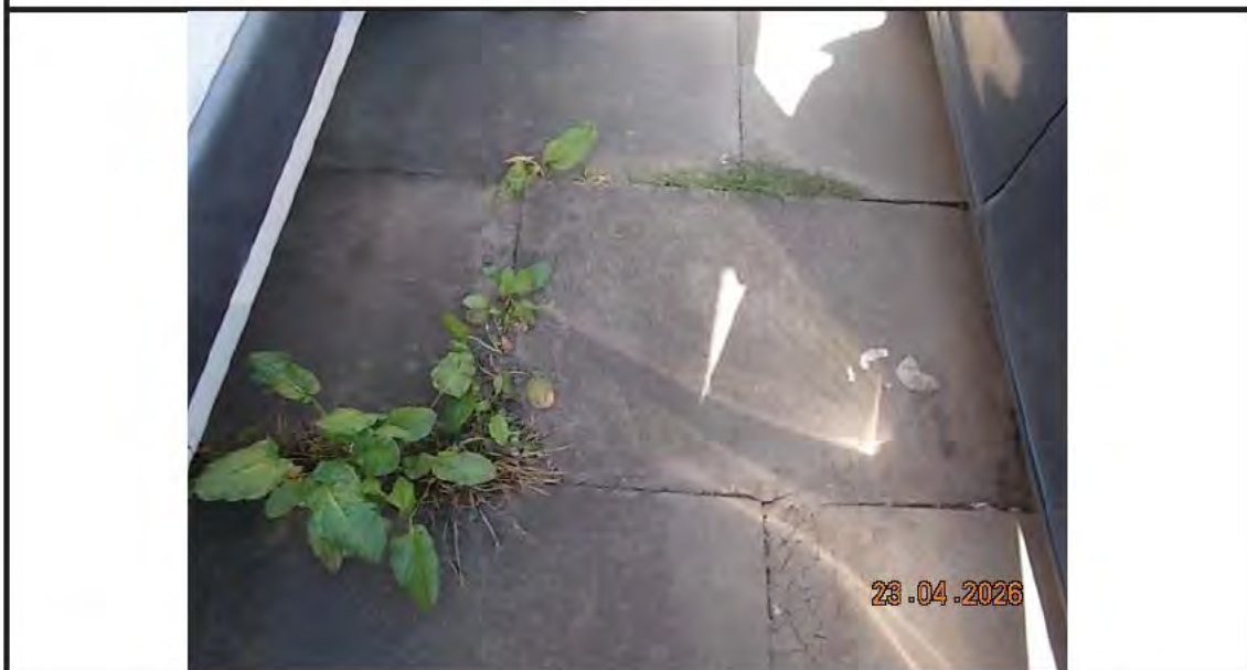
24. Driveway to front of House
