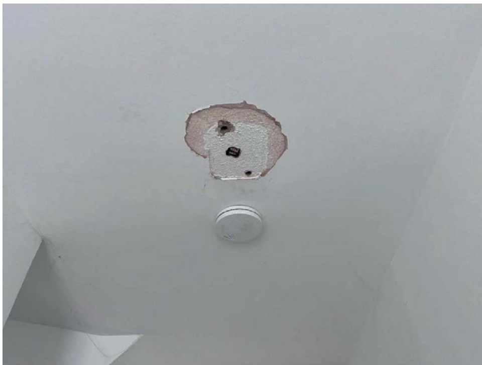
Smoke detector on Hall ceiling.
