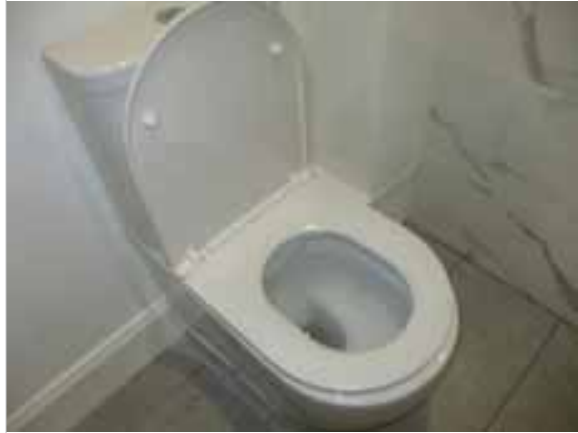
Shower Room - new toilet
