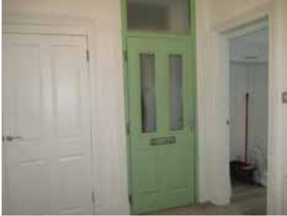
Front door - adjustments carried out, new lock installed and re-painted
