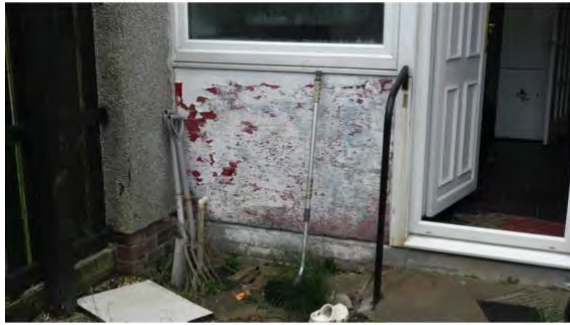
Photo 8 – Exposed plywood on rear elevation
