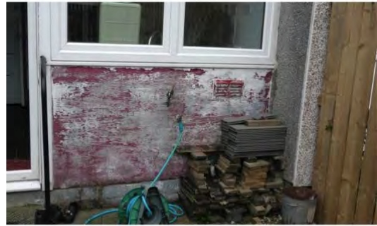
Photo 9 – Exposed plywood on rear elevation
