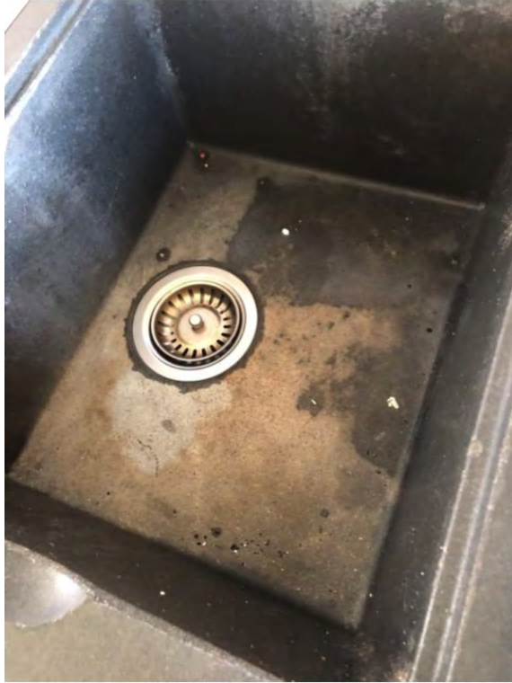
Photo 14 – Fixed sink basin in kitchen
