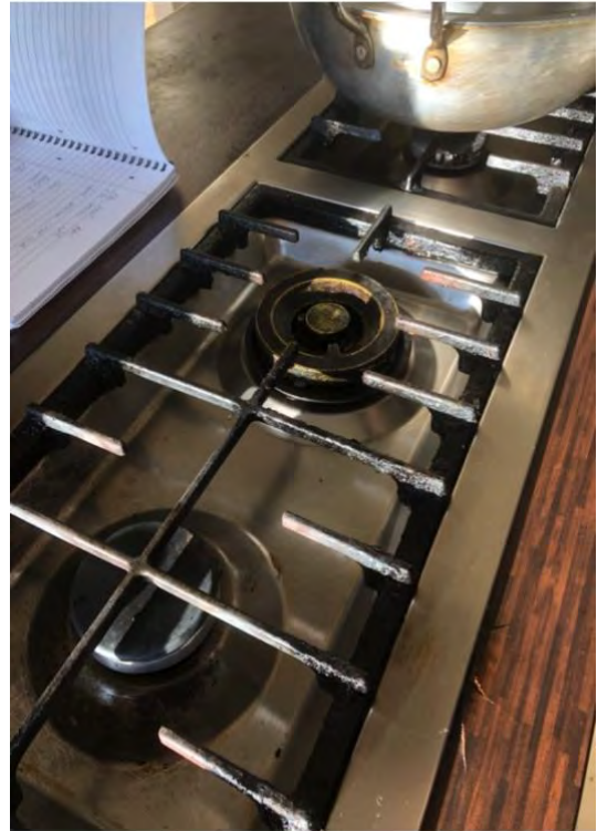
Photo 11 – Broken/part-missing gas hob ring
