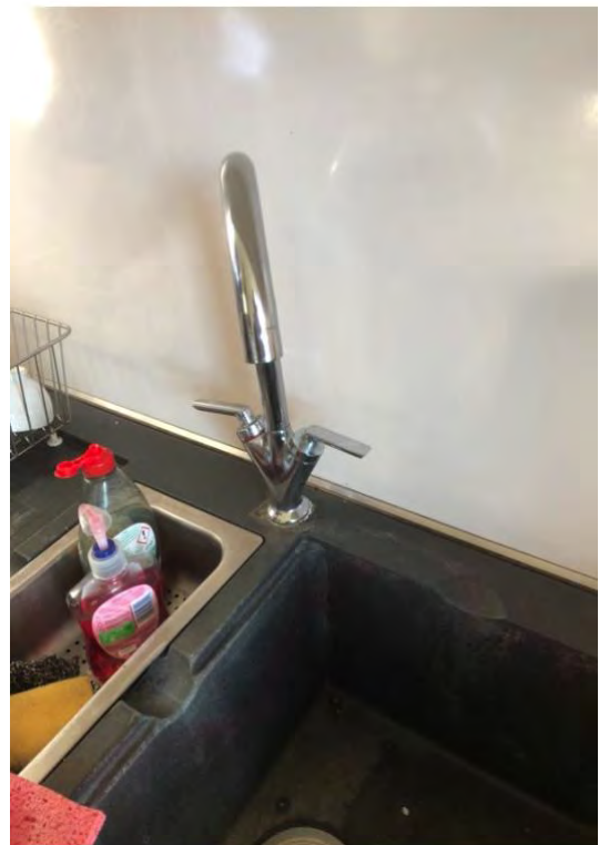
Photo 13 – Replaced mixer tap in kitchen
